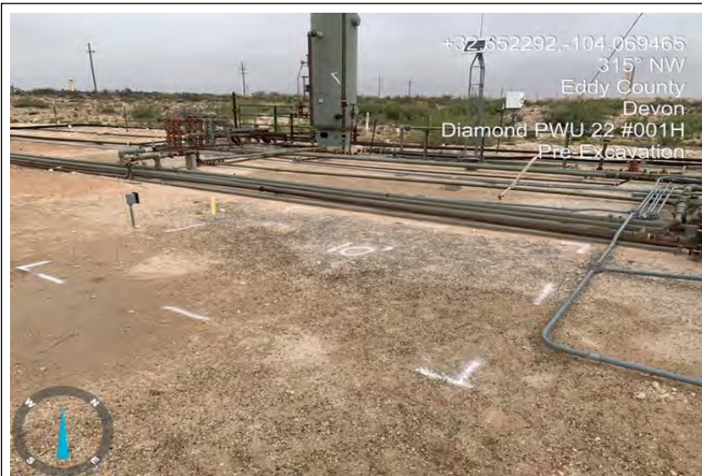
Flagging/marking excavation area
