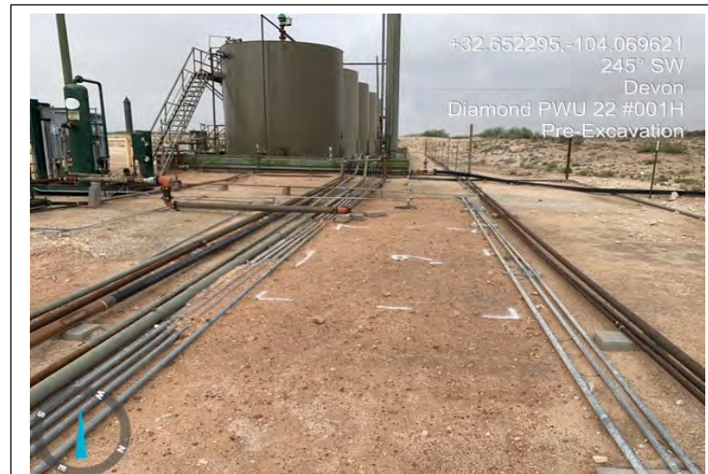
Flagging/marking excavation area
