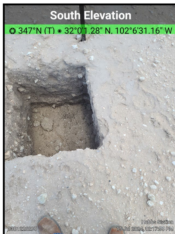
View of historical release extent after hydro-excavation delineation activities, facing north (07/15/24).
