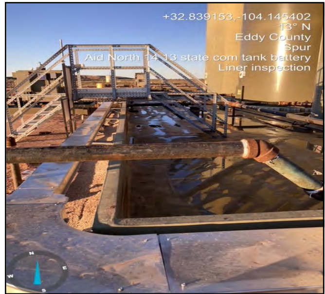
Photo of liner pursuant to being power washed facing North. Fluid from power washer.
