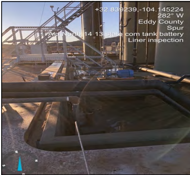
Photo of liner pursuant to being power washed facing West. Fluid from power washer
