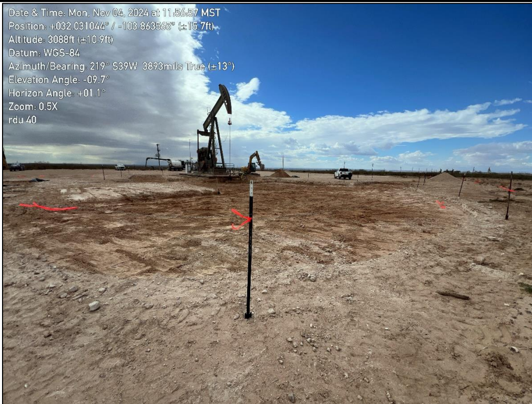
PHOTO 8: Southwestern view of excavation extent. 11/04/2024
