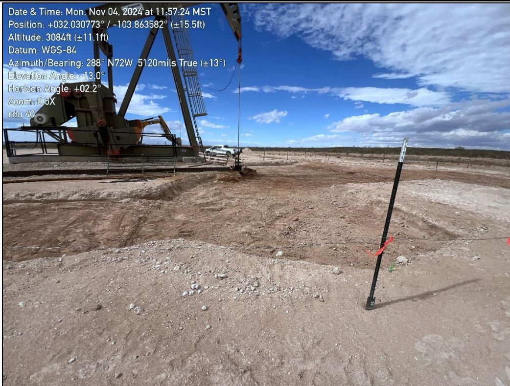
PHOTO 7: Northwestern view of excavation extent. 11/04/2024
