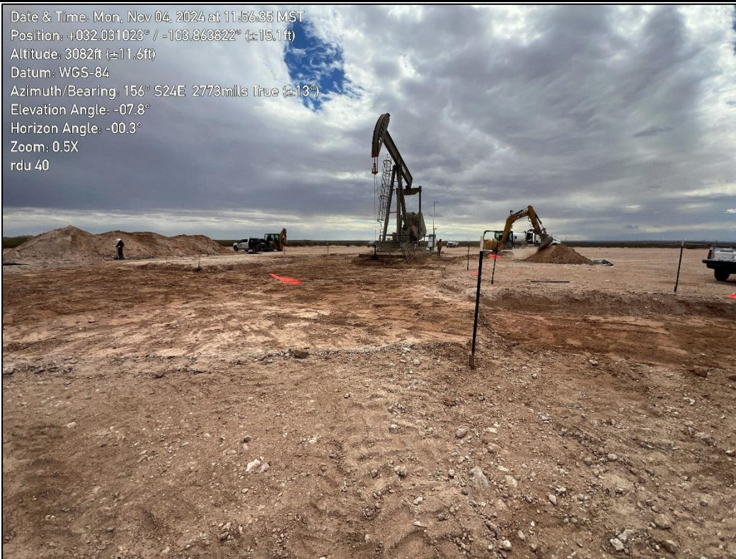
PHOTO 6: Southeastern view during excavation activities. 11/04/2024
