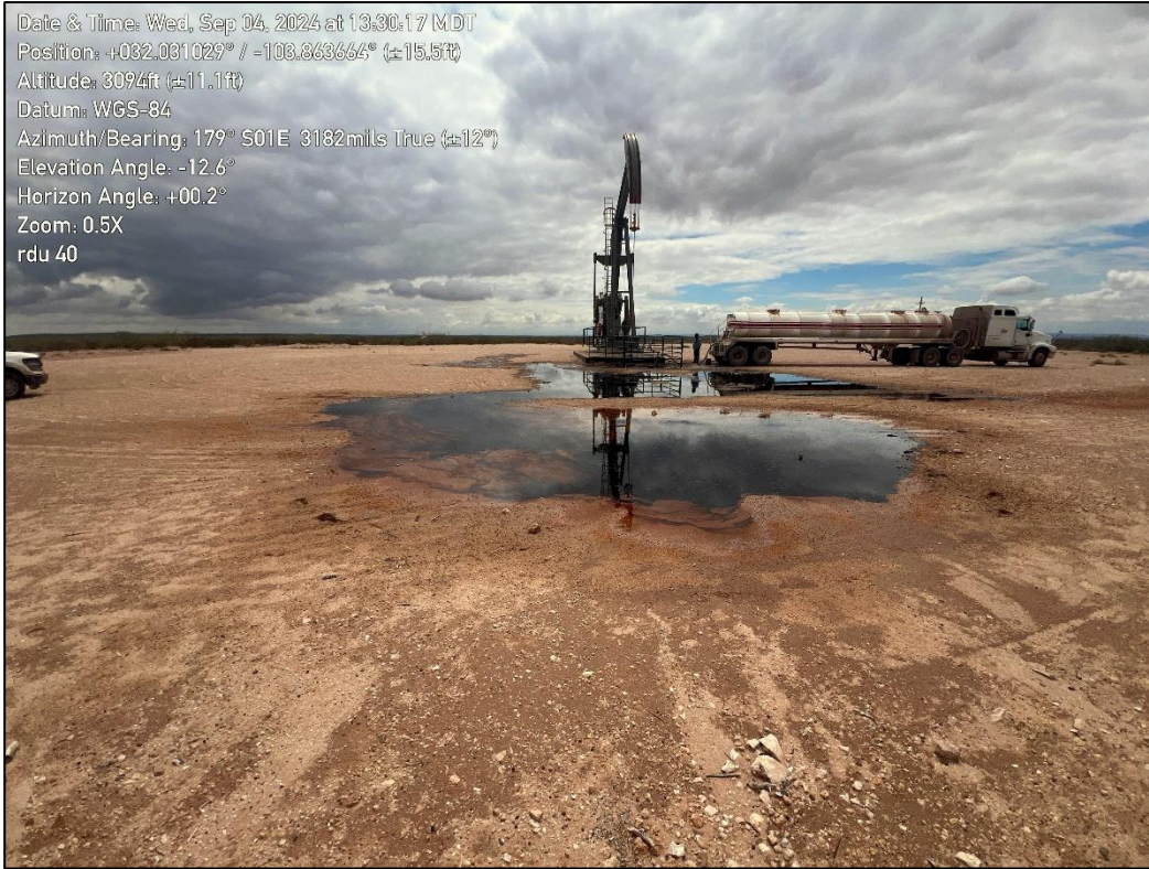
PHOTO 1: Southeastern view during initial site assessment. 09/04/2024
