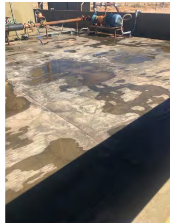
Figure 2. View of the Inspected Liner.
