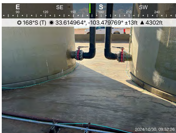
Figure 5. View of the Inspected Liner.
