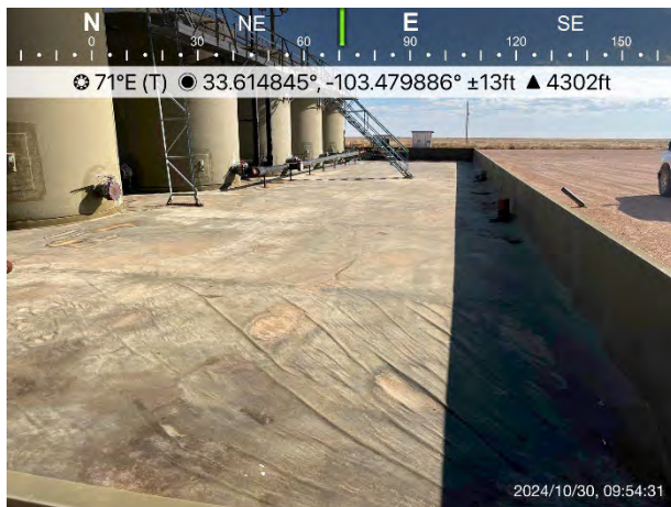
Figure 3. View of the Inspected Liner.
