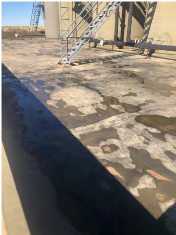
Figure 1. View of the Inspected Liner.
