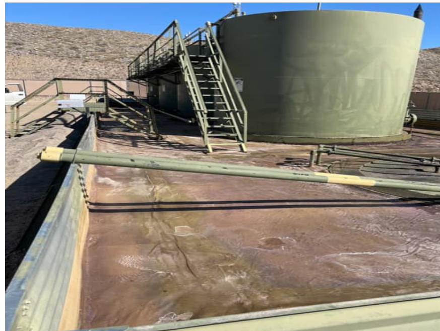
Photograph 2 (dated 10/10/2024) – View looking N at secondary containment with the liner exposed.
