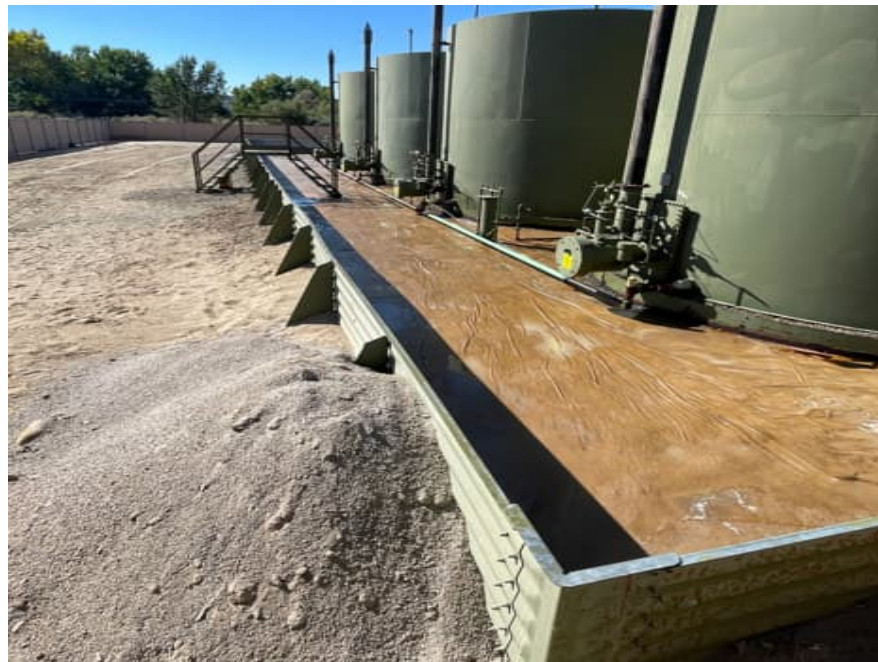
Photograph 3 (dated 10/10/2024) – View looking SW at the exposed liner within secondary containment.
