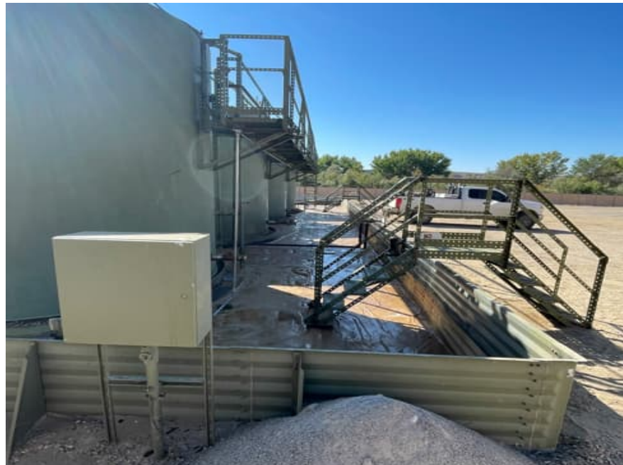
Photograph 4 (dated 10/10/2024) – View looking S at the exposed liner within secondary containment.
