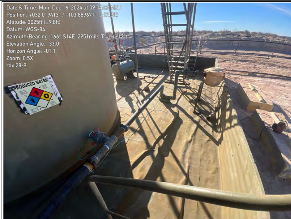
PHOTO 3: Southeast view of the lined secondary containment during liner inspection. 12/16/2024
