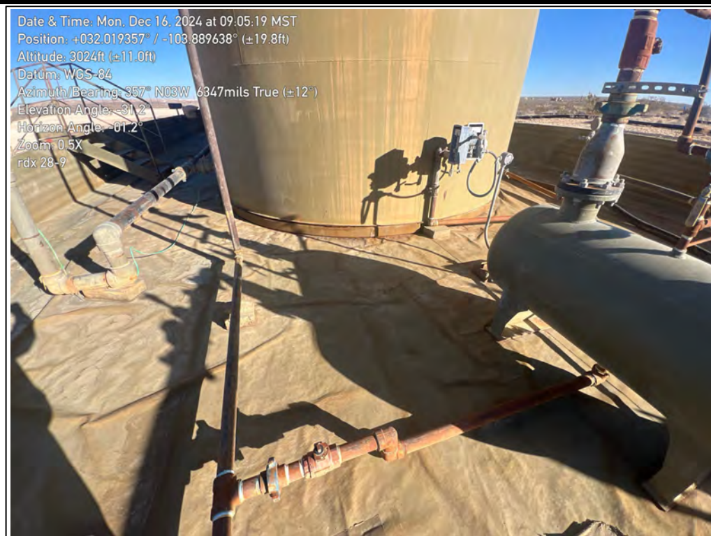
PHOTO 4: Northwest view of the lined secondary containment during liner inspection. 12/16/2024
