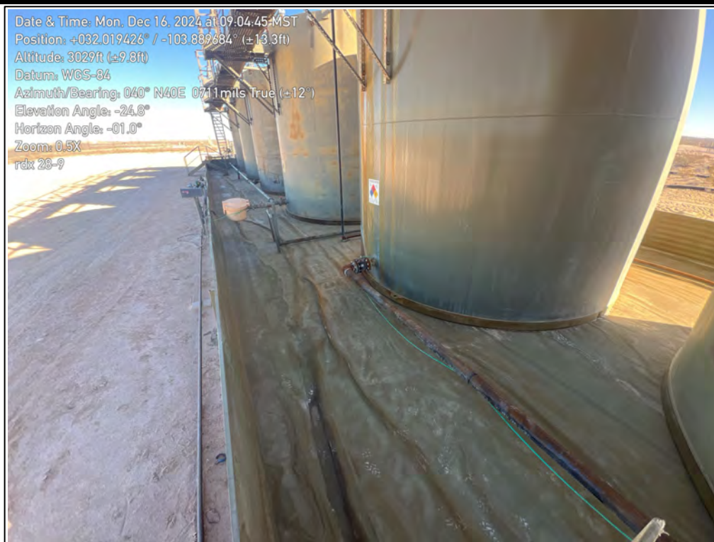
PHOTO 2: Northeastern view of the lined secondary containment during liner inspection. 12/16/2024
