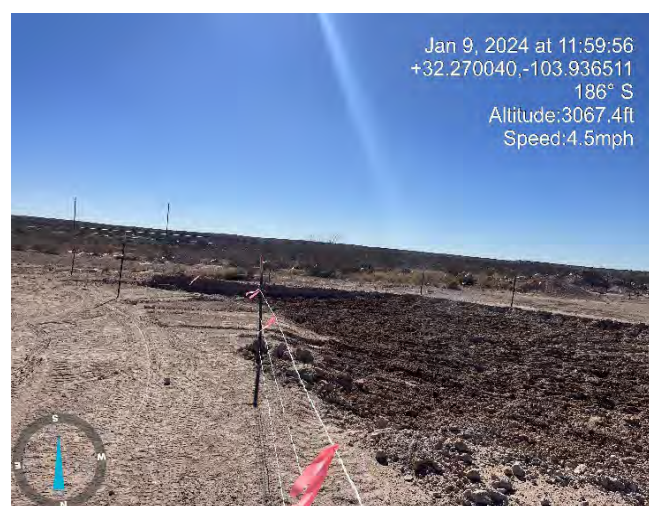
Photograph 3 Date: 01/09/2024 Description: Excavation activities View: South
