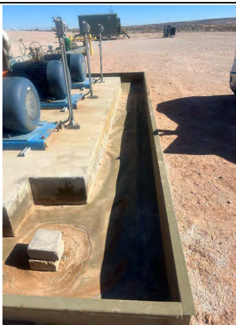
Photograph 3 Date: 01/13/2023 Description: Liner inspection activities. View: East
