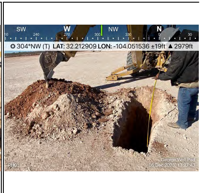
Photograph 4 Date: 12/05/2023 Description: PH03; Vertical Delineation Sampling View: Northwest
