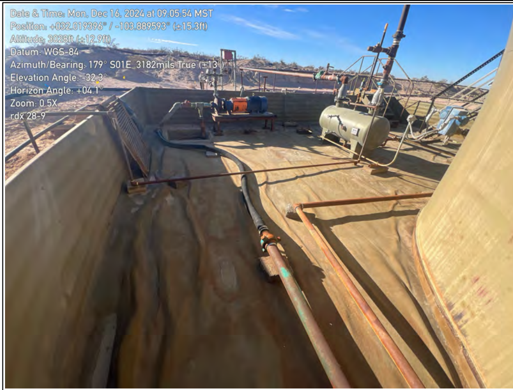
PHOTO 5: Southeast view of the lined secondary containment during liner inspection. 12/16/2024
