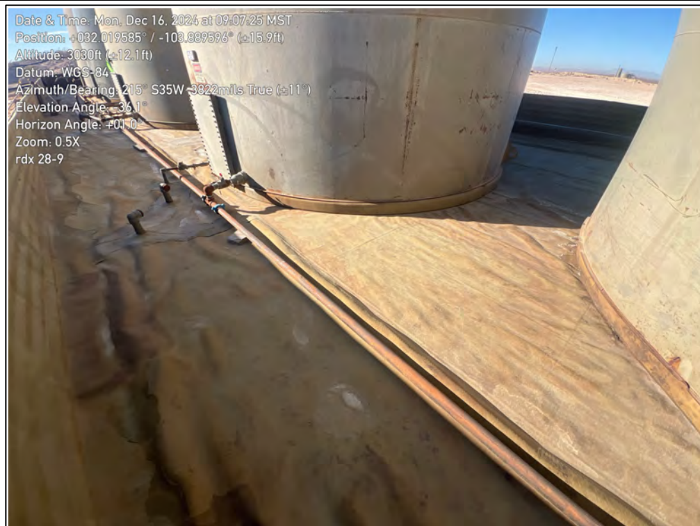
PHOTO 8: Southwest view of the lined secondary containment during liner inspection. 12/16/2024
