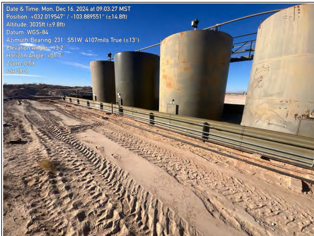
PHOTO 10: Southwest exterior view of the lined secondary containment during liner inspection. 12/16/2024
