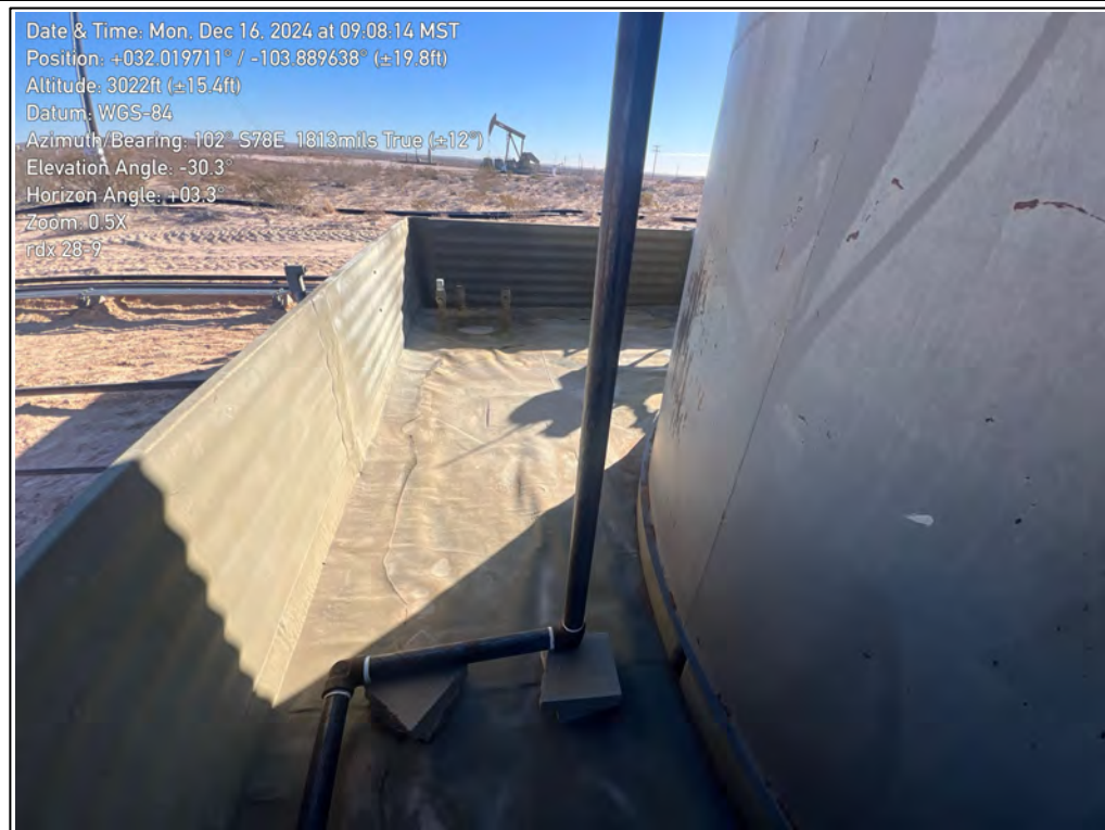
PHOTO 6: Southeast view of the lined secondary containment during liner inspection. 12/16/2024
