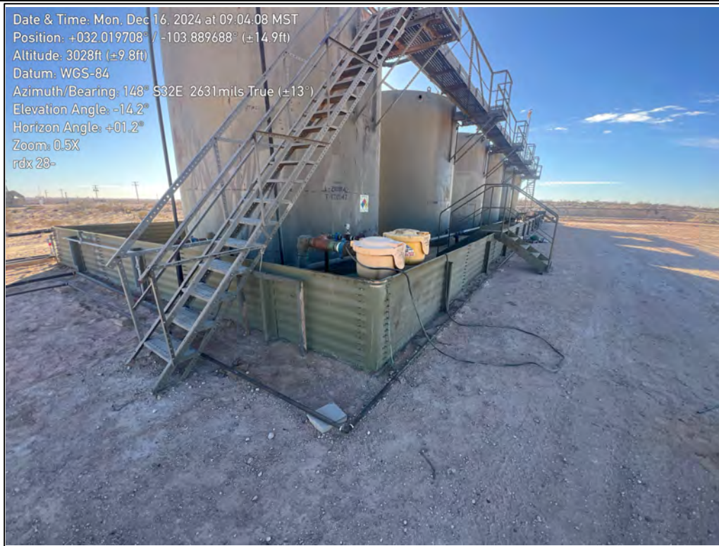
PHOTO 11: Southeast exterior view of the lined secondary containment during liner inspection. 12/16/2024
