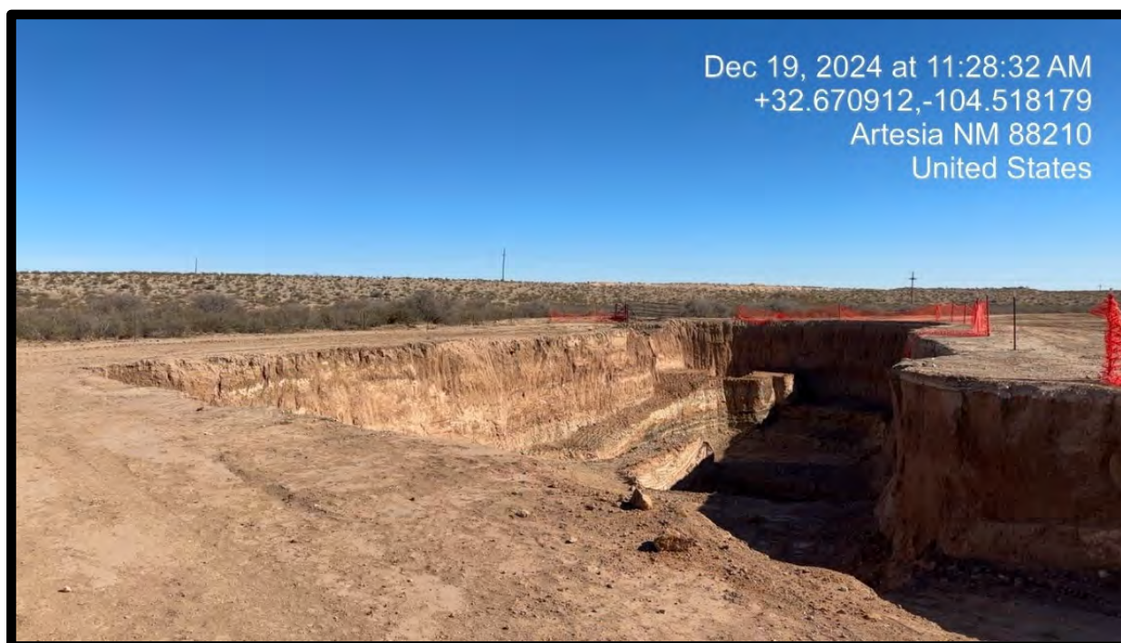
PHOTOGRAPH NO. 3 – A view of the Tank Battery Area upon completion. The view is towards the northeast.
