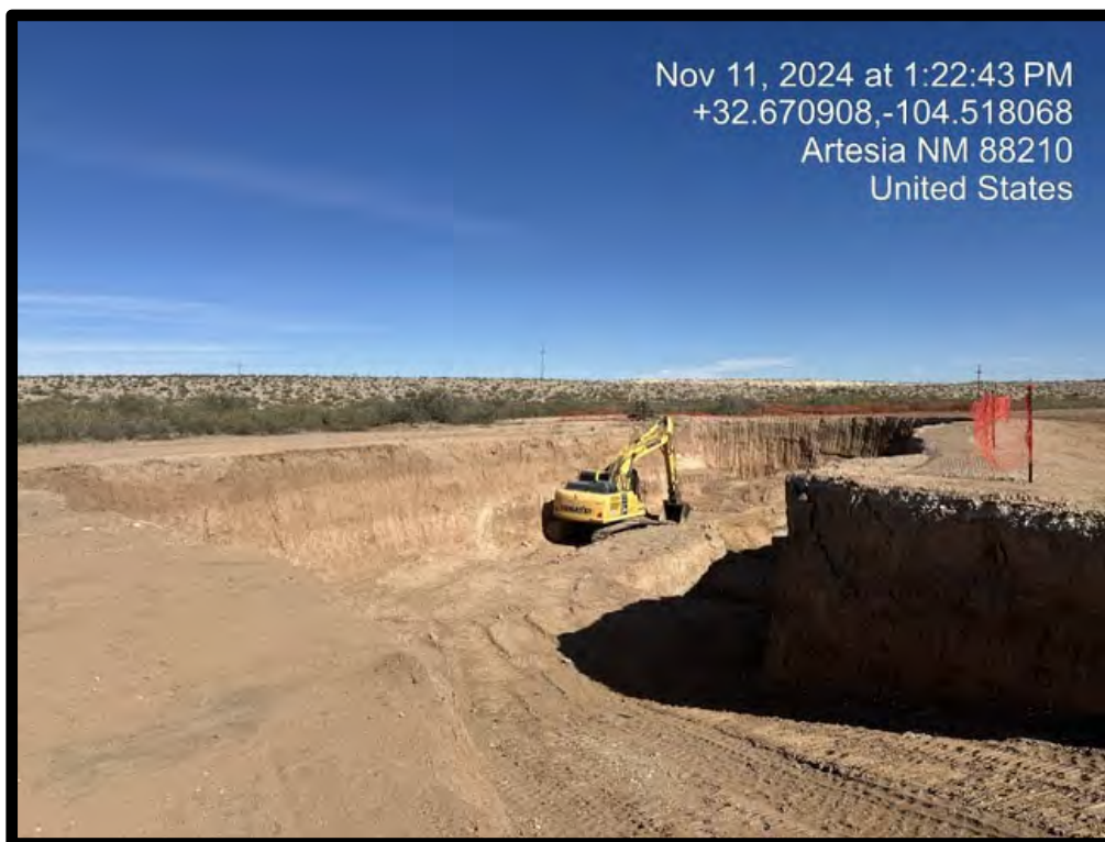
PHOTOGRAPH NO. 2 – A view of the Tank Battery Area during the soil removal operations. The view is towards the northeast.
