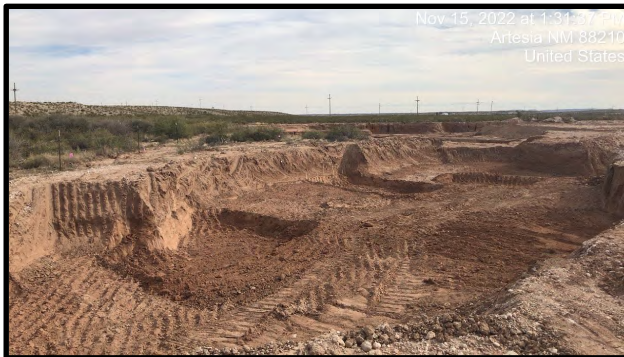
PHOTOGRAPH NO. 4 – A view of the “Eastern” Pad Area during the remediation process. The view is towards the southeast.
