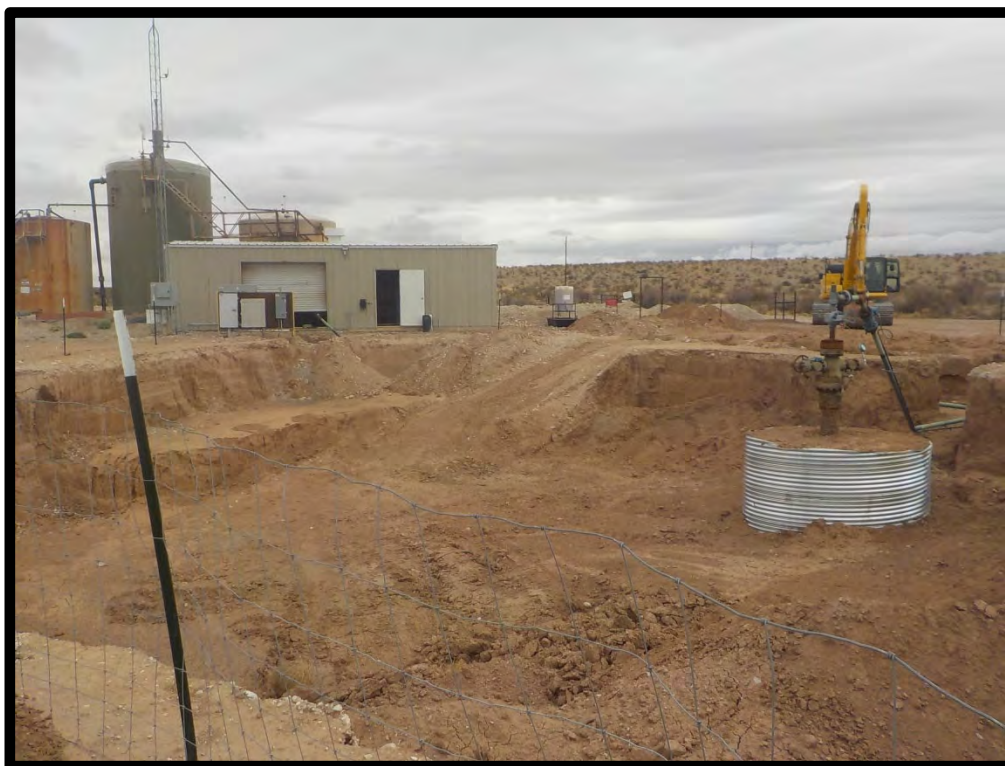
PHOTOGRAPH NO. 1 – A view of “Wellhead Area” during the soil removal and preparation process. The view is towards the northeast.
