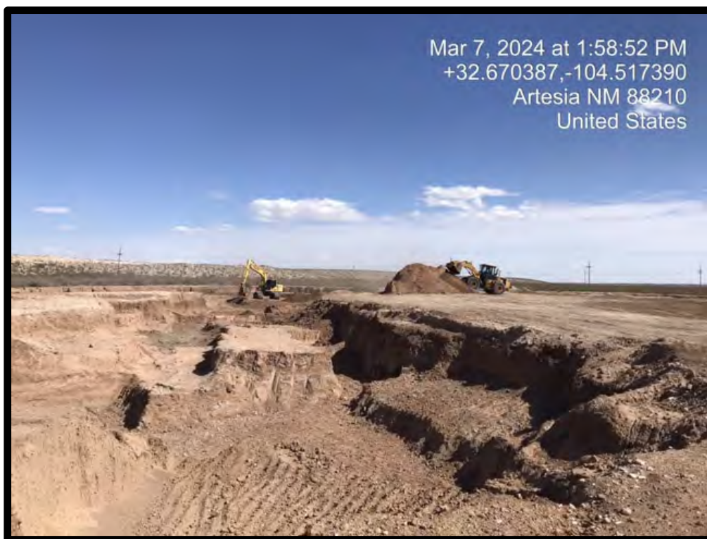
PHOTOGRAPH NO. 9 – A view “Southern” Pad Excavation Area upon completion. The view is towards the south.
