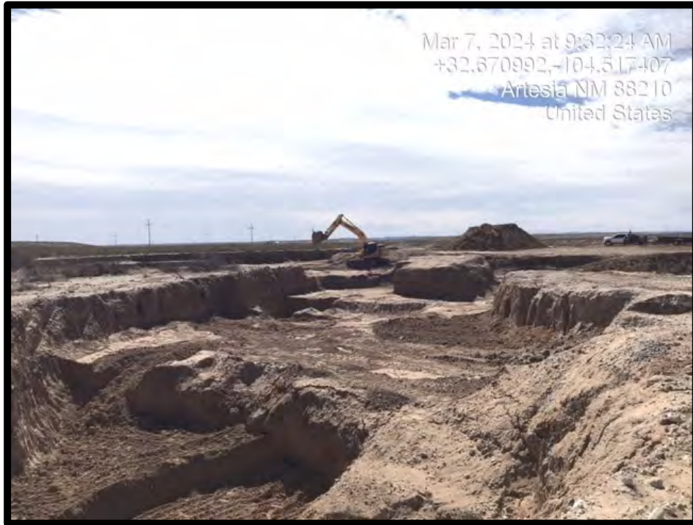
PHOTOGRAPH NO. 7 – A view “Eastern” Pad Excavation Area upon completion. The view is towards the east.
