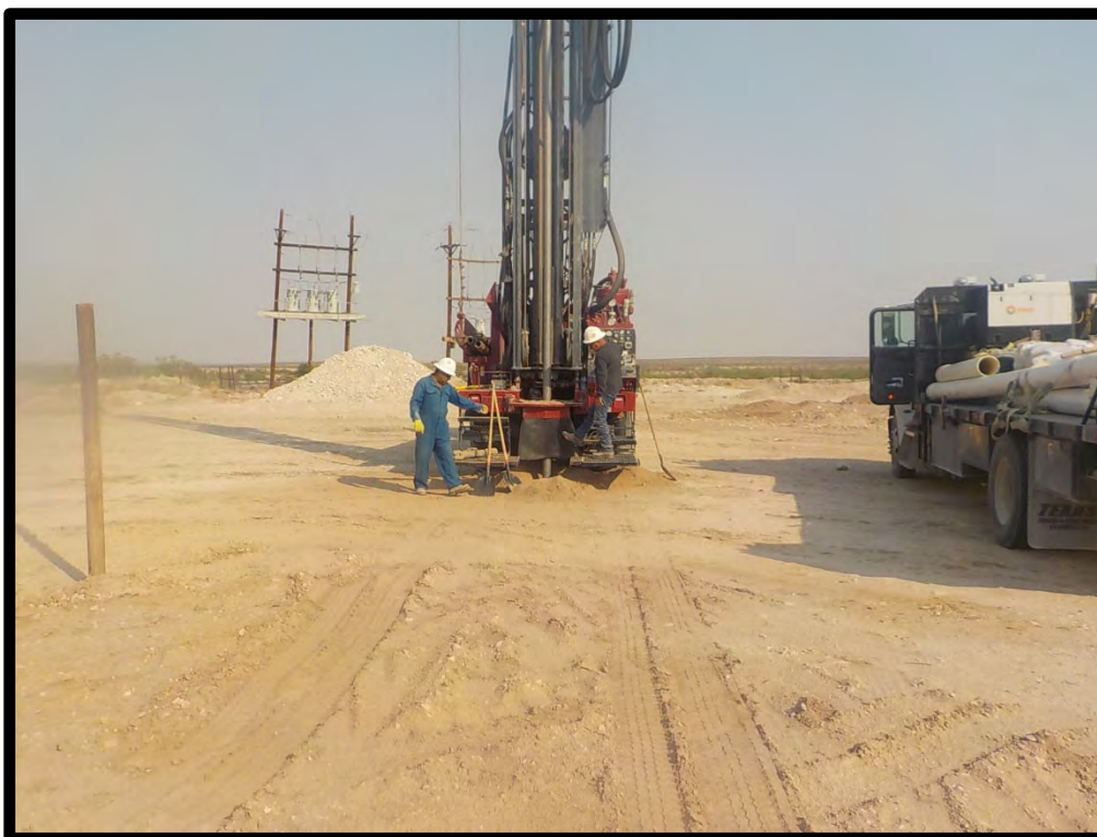
PHOTOGRAPH NO. 3 – A view of vertical delineation soil boring activities in the “Wellhead Area” on May 19, 2022. The former Roy SWD #3 well head location can be seen in the left-hand side of the photograph. The view is towards the northwest.
