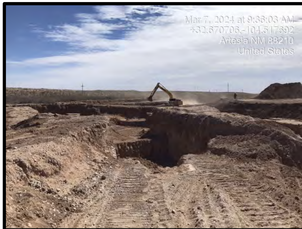
PHOTOGRAPH NO. 8 – A view “Middle” Pad Excavation Area upon completion. The view is towards the east.
