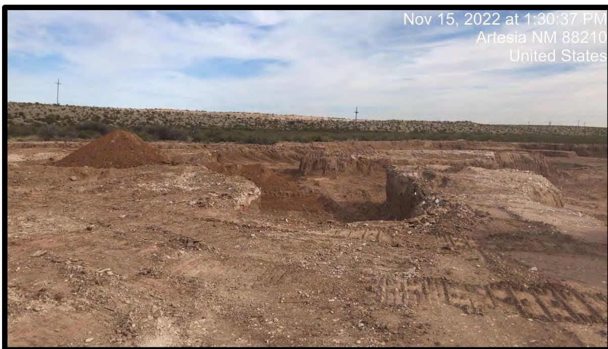
PHOTOGRAPH NO. 5 – A view of the “Middle” Pad Area during the remediation process. The view is towards the east.
