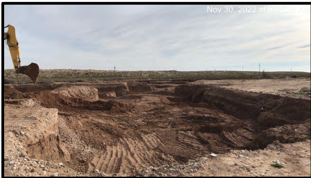
PHOTOGRAPH NO. 6 – A view of the “Southern” Pad Area during the remediation process. The view is towards the east.
