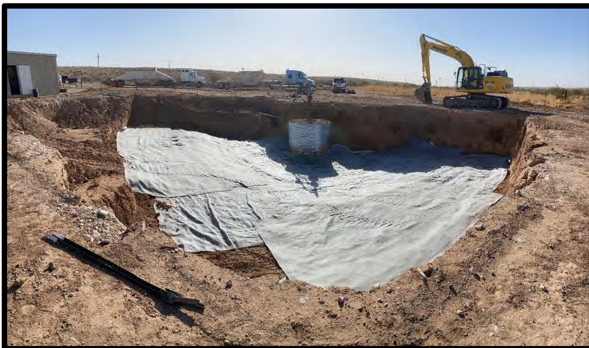
PHOTOGRAPH NO. 2 – A view of the “Wellhead Area” during the GCL installation process in April 2022. The view is towards the southeast.
