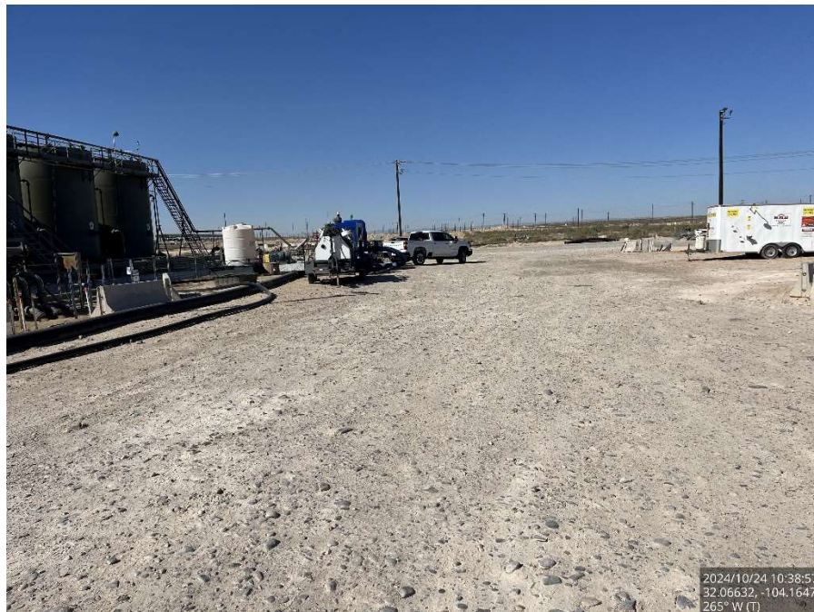
Area impacted by release on the pad, viewing to the west.
