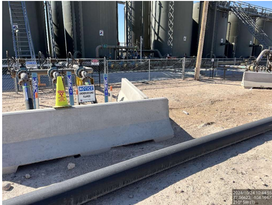
Area impacted by release on the pad, viewing to the southwest.
