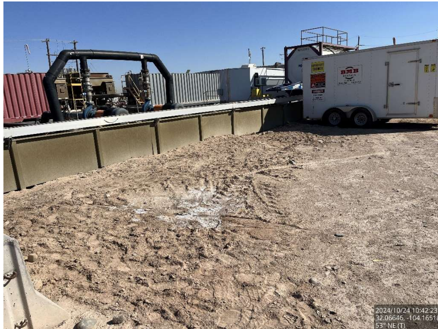
Area impacted by release on the pad, viewing to the northeast.
