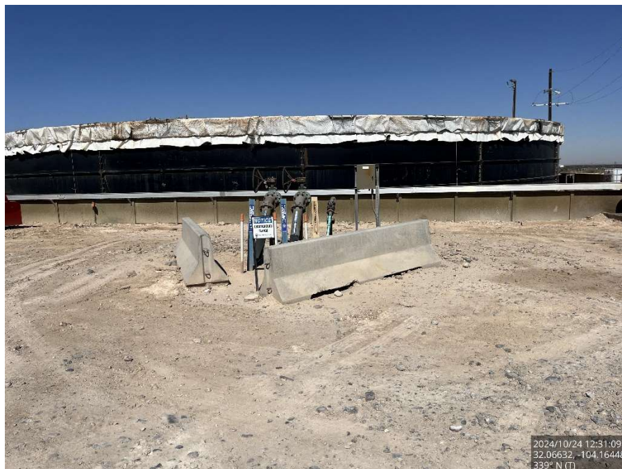
Area impacted by release on the pad, viewing to the north.
