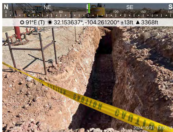
Figure 10. View of the excavation.
