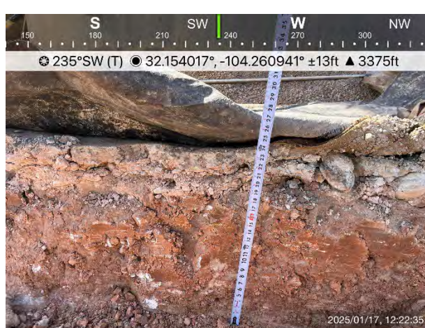
Figure 12. Excavation depth verification.
