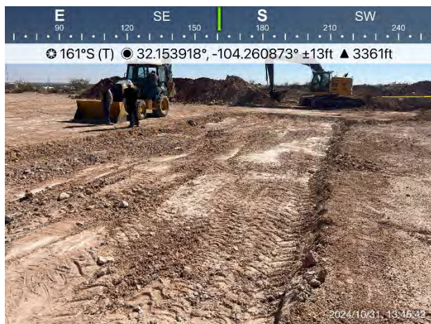
Figure 1. View of the excavation.
