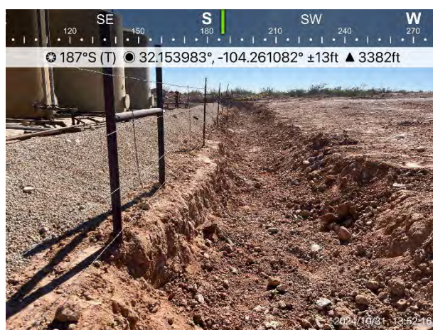
Figure 6. View of the excavation.
