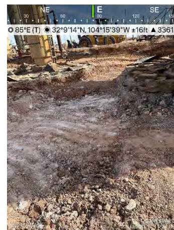
Figure 22. View of the excavation.
