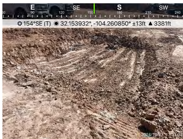
Figure 4. BS-08 - 1.5 ft area of the excavation.
