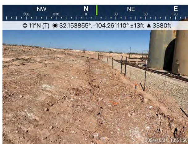
Figure 8. View of the excavation.
