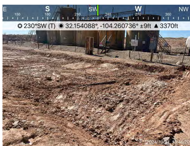
Figure 2. View of the excavation.
