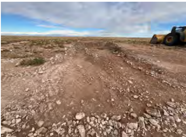
View to E of excavation (11/4/24).
