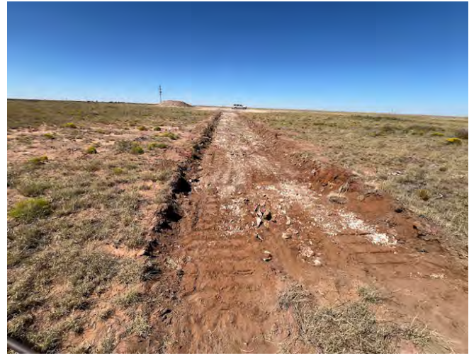
View to W of excavation (9/26/24).
