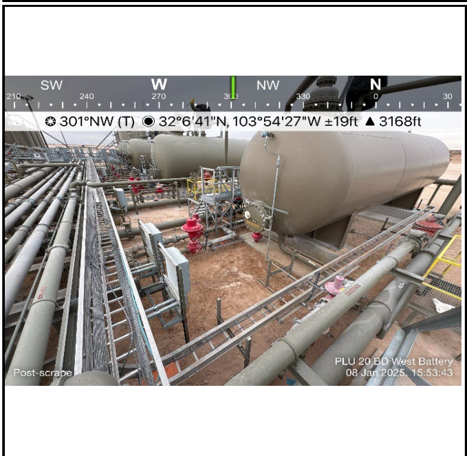
Photograph: 4 Date: 1/8/2025 Description: Surface scraping activities View: Northwest
