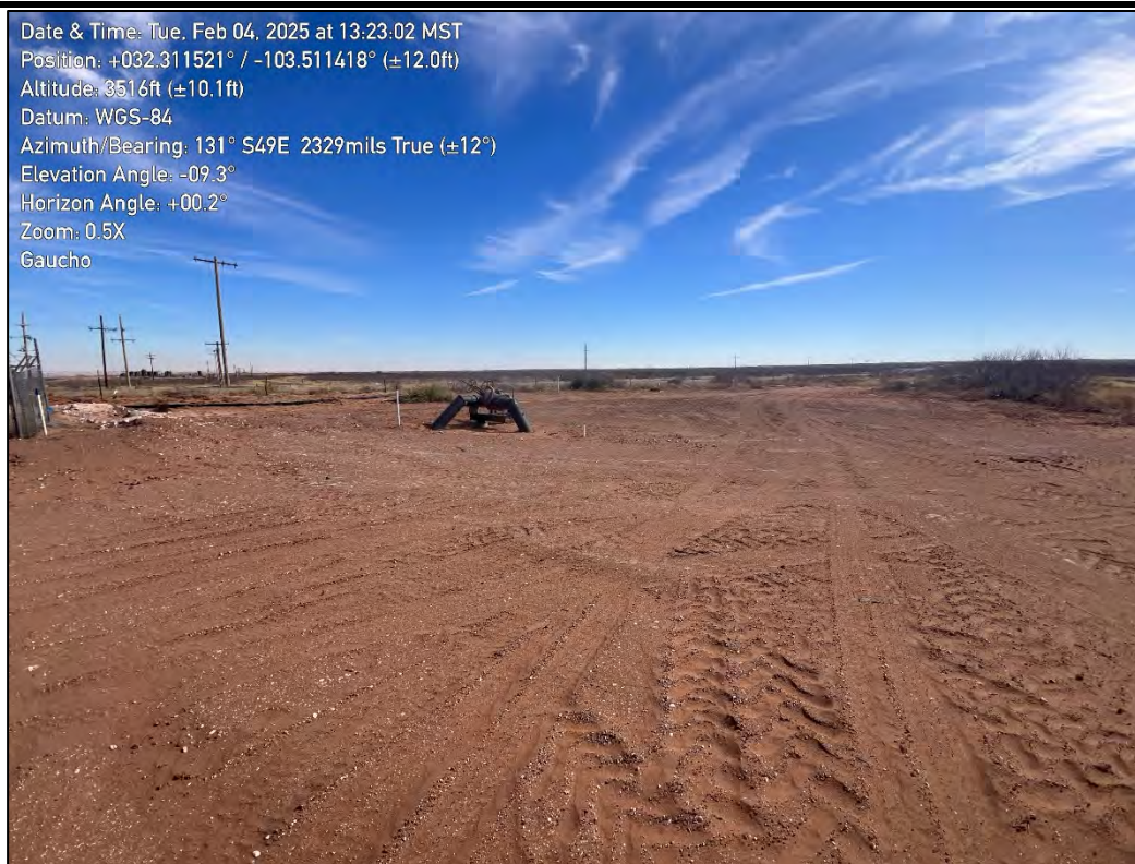
PHOTO 10: Southeastern view following restoration activities. 02/04/2025
