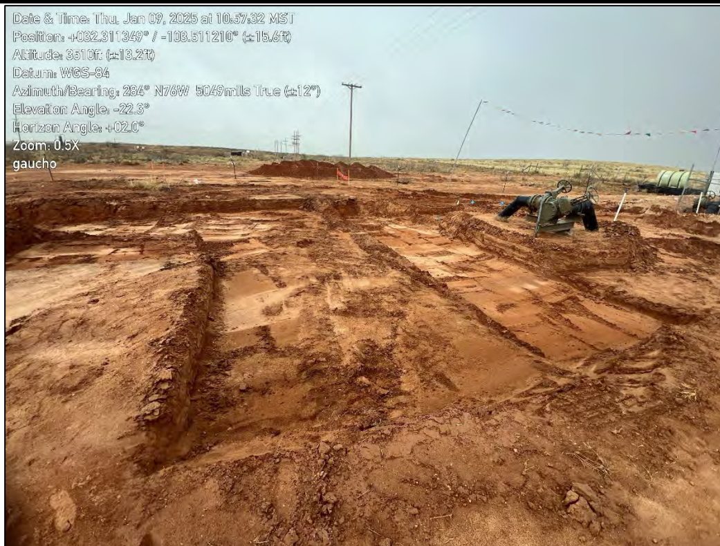
PHOTO 9: Northwestern view of final Excavation Extent. 01/09/2025
