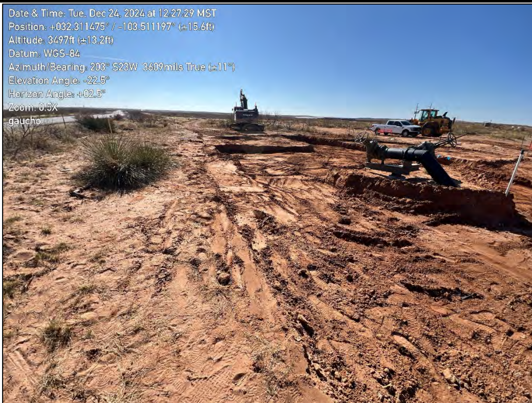
PHOTO 7: Southwestern view during excavation activities. 12/24/2024
