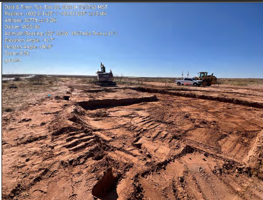
PHOTO 6: Southwestern view during excavation activities. 12/24/2024
