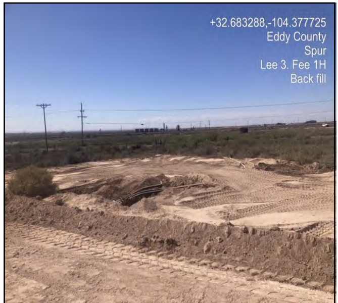
Photograph of the excavation being backfilled and completed prior to seeding.
