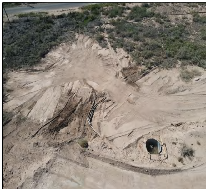
Photograph taken from a drone of the excavation being backfilled and completed prior to seeding.
