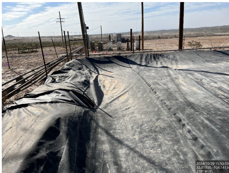
Repaired liner on southside of battery, viewing to the west.
