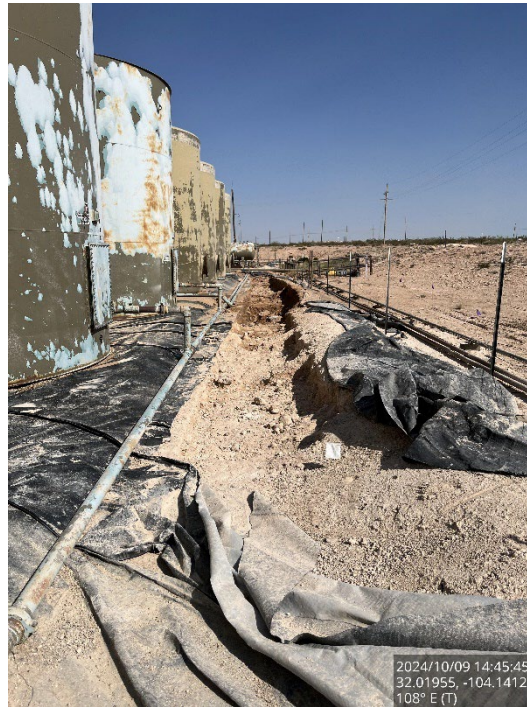
Hydro-excavated area on the south side of tank battery, viewing to the east.
