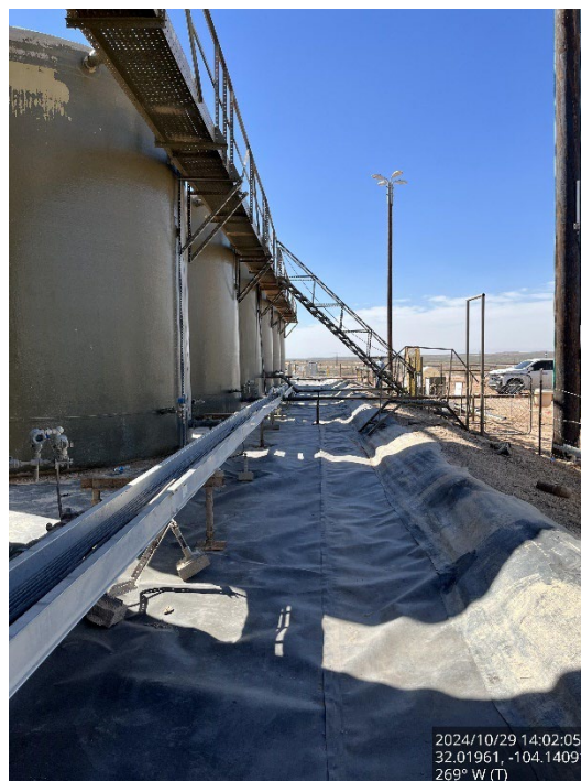
Repaired liner on north side of battery, viewing to the west.
