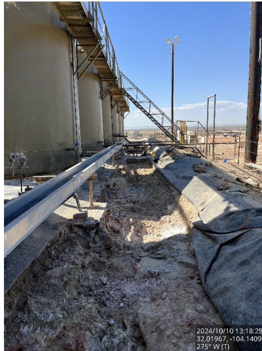
Hydro-excavated area on the north side of tank battery, viewing to the west.
