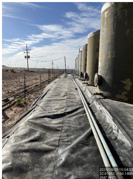
Repaired liner on southside of battery, viewing to the west.
