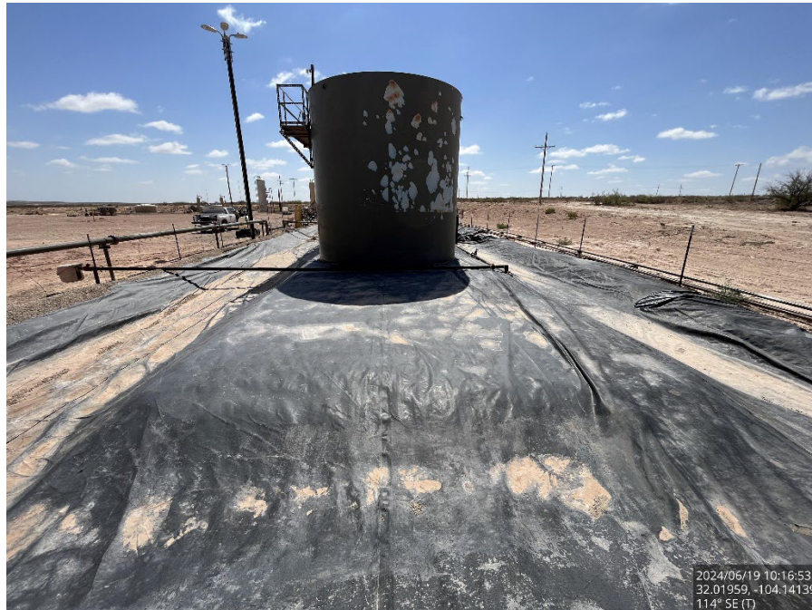
Lined tank battery containment where release occurred, viewing to the southeast.
