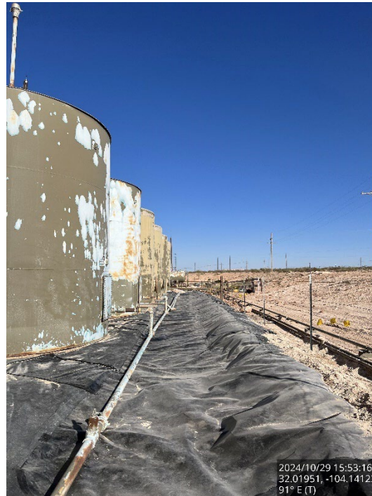
Repaired liner on south side of battery, viewing to the east.
