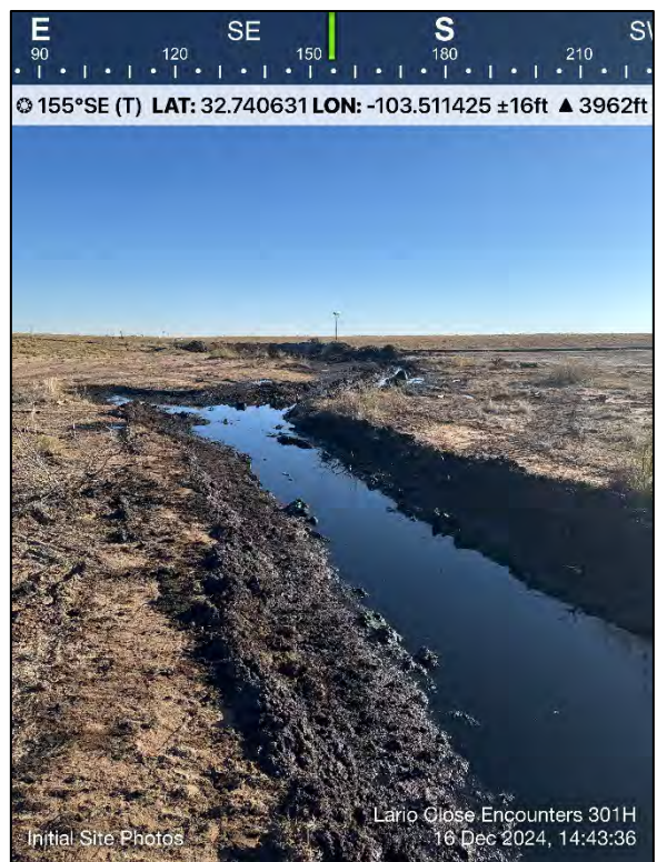
Photo 14: Initial site conditions, Iron House Draw
