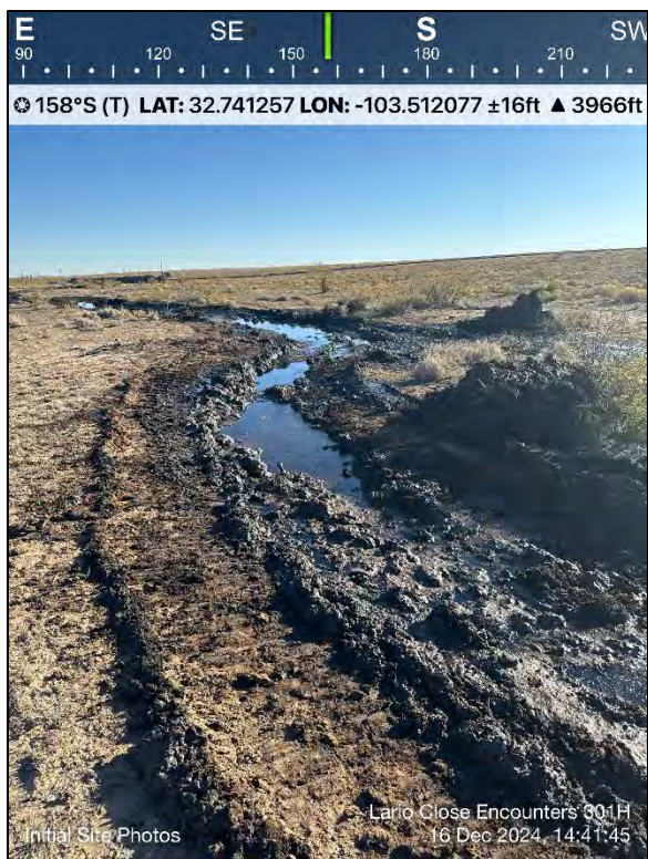
Photo 13: Initial site conditions, Iron House Draw
