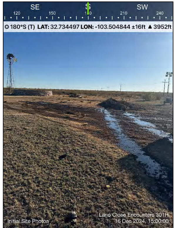
Photo 18: Initial site conditions, terminus of release
