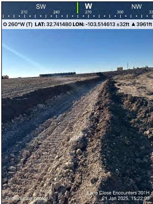
Photo 23: Remediation progress, wash east of pad
