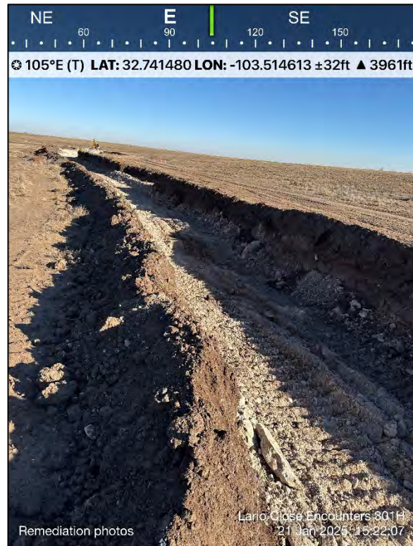
Photo 24: Remediation progress, wash east of pad
