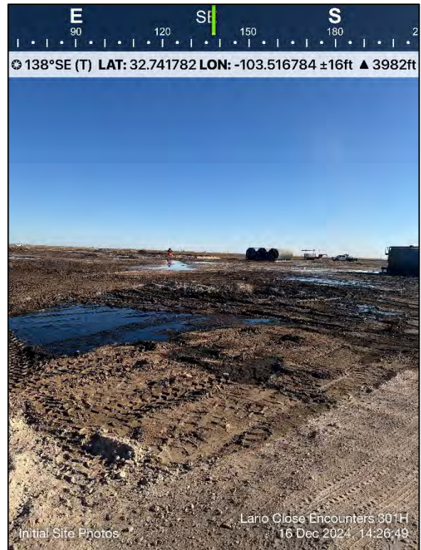
Photo 2: Initial site conditions, drilling Pad
