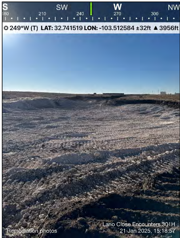
Photo 25: Remediation progress, Iron House Draw
