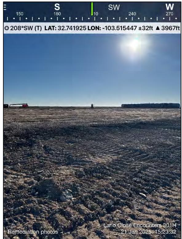
Photo 22: Remediation progress, drilling pad
