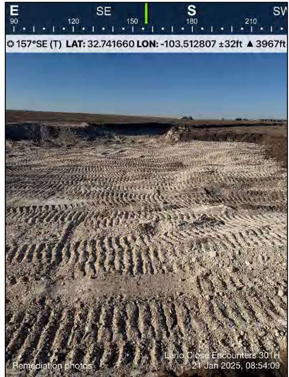
Photo 30: Remediation progress, Iron House Draw
