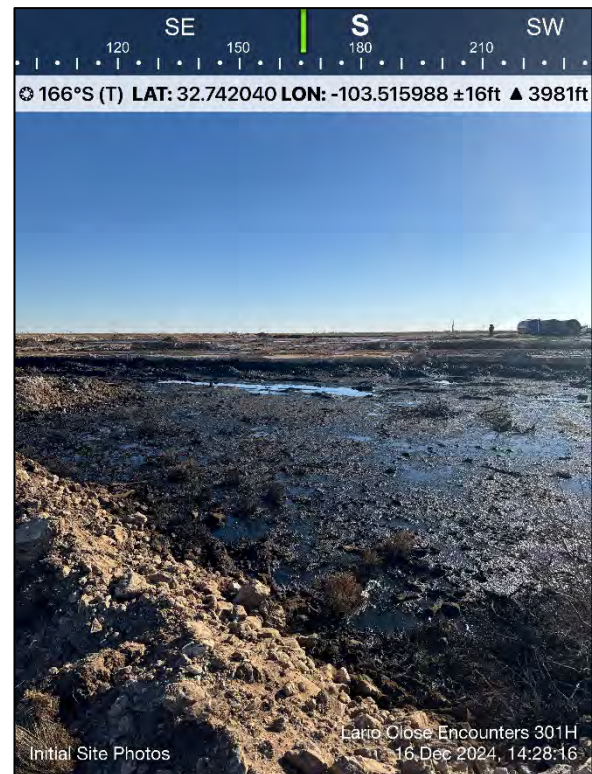
Photo 4: Initial site conditions, north of drilling pad
