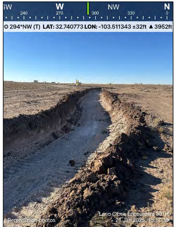
Photo 26: Remediation progress, Iron House Draw
