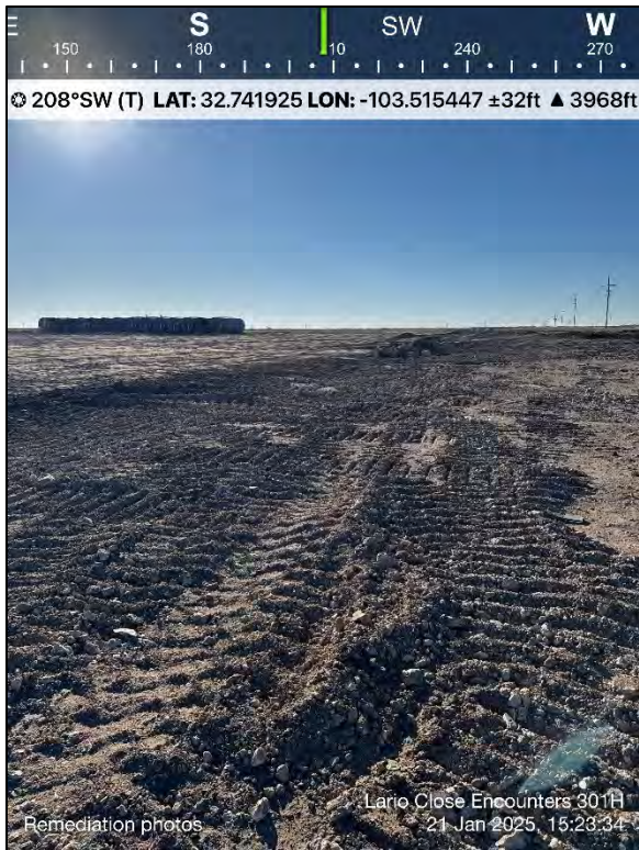
Photo 21: Remediation progress, drilling pad
