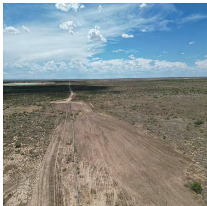
Site Retored to Grade.
