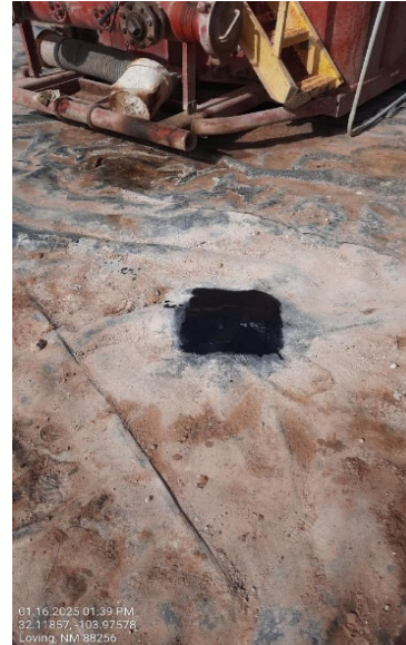
Photograph: 2 Date: 01/16/2025 Description: Patched Liner View: Direct
