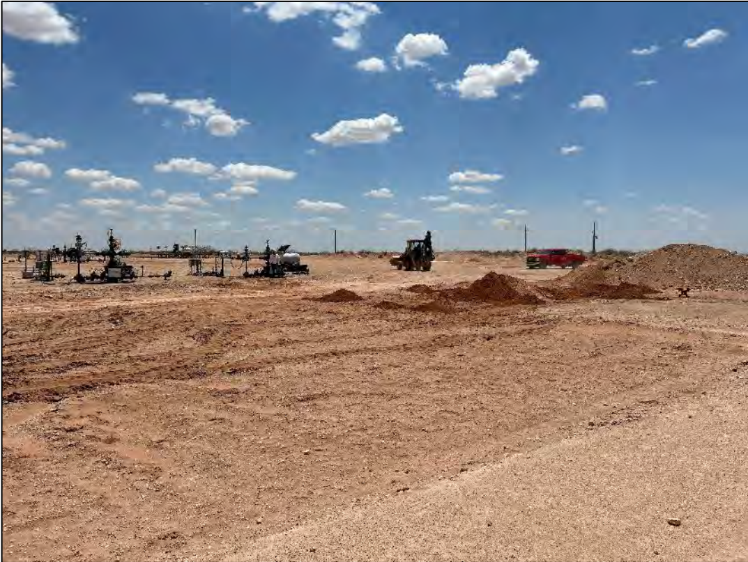
PHOTO 8: View of the excavated area facing southwest. 07/09/2024
