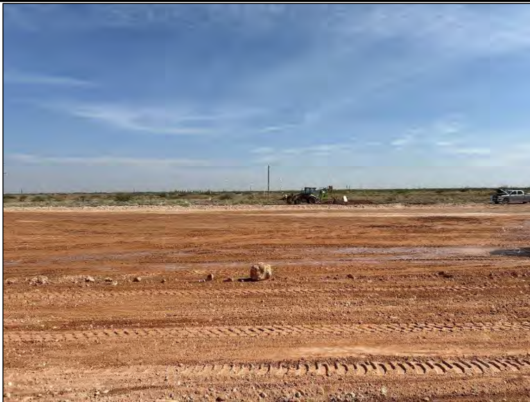
PHOTO 13: View of the remediated area facing north. 08/02/2024
