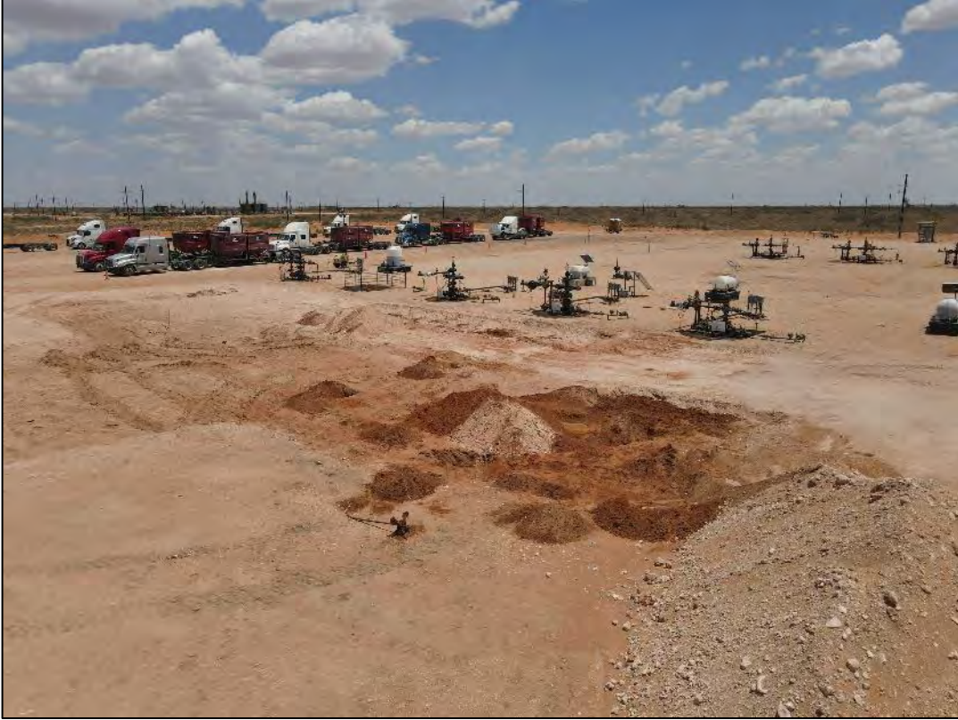
PHOTO 7: View of the excavated area facing southeast. 07/09/2024
