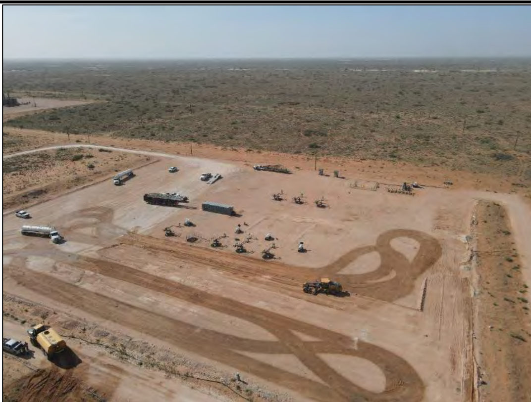
PHOTO 12: View of the impacted area facing southeast. 08/02/2024
