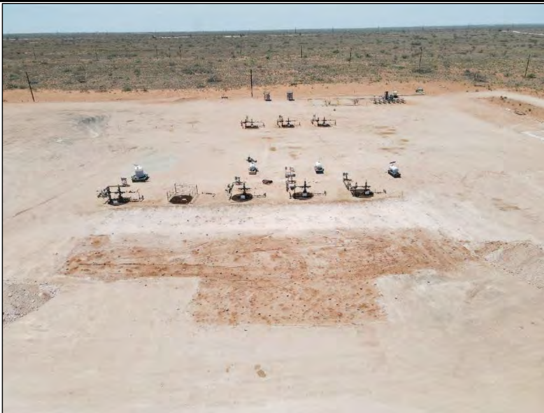
PHOTO 5: View of the excavated area facing south. 06/26/2024
