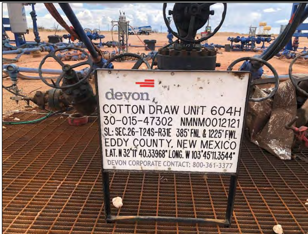
PHOTO 1: View of the impacted areas sign facing south. 8/30/22
