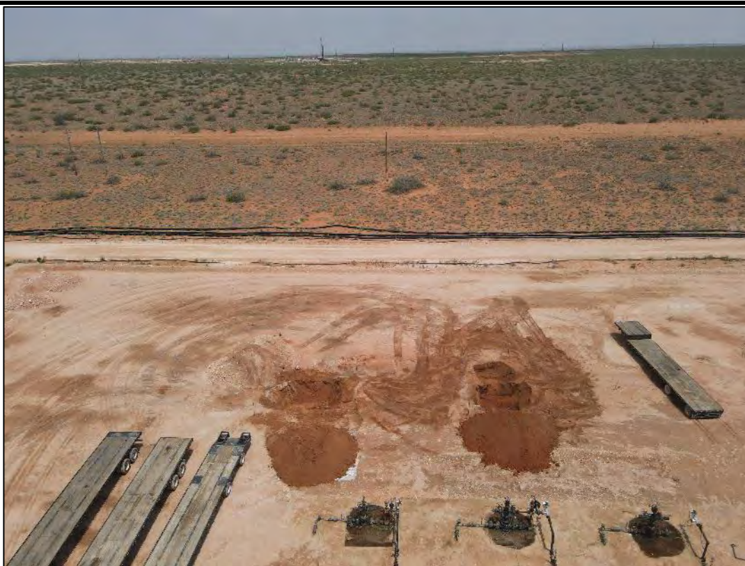
PHOTO 10: View of the impacted area facing north. 07/23/2024
