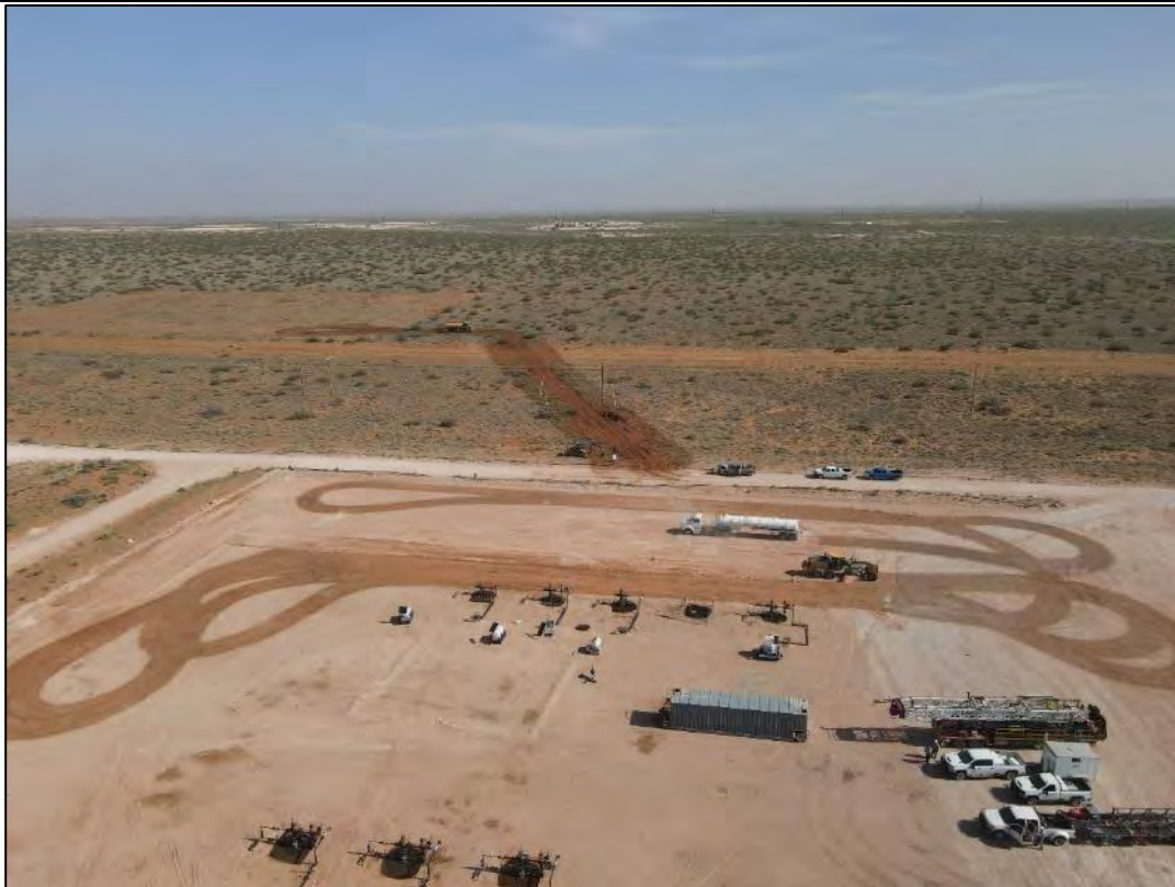
PHOTO 11: View of the remediated area facing north. 08/02/2024
