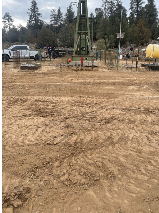
Photo 15: Excavated areas have been backfilled with clean material, 1/6/2025.
