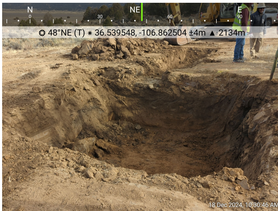
Photo 5: Wellhead excavation and new release excavation.
