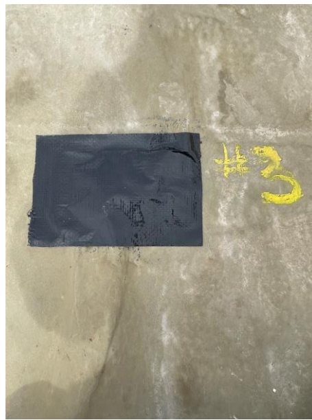
Liner Sample Point #3-patched
