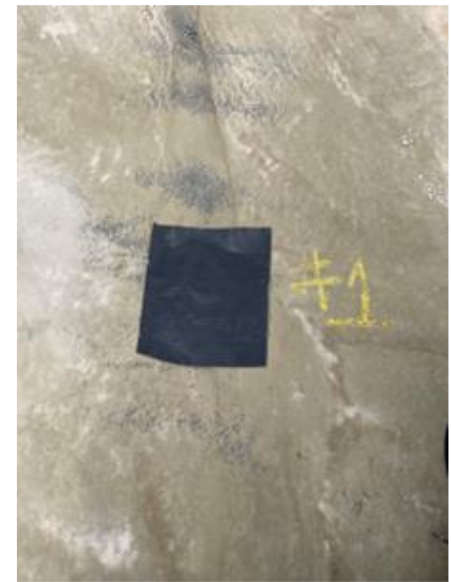
Liner Sample Point #1-patched
