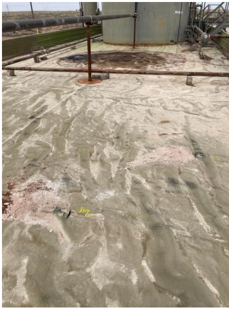
Liner Sample Point #1-facing North
