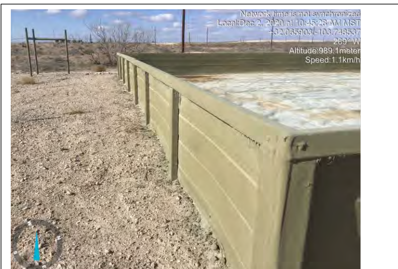
Southeast corner facing West outside
