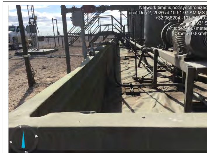
Northeast corner facing South inside
