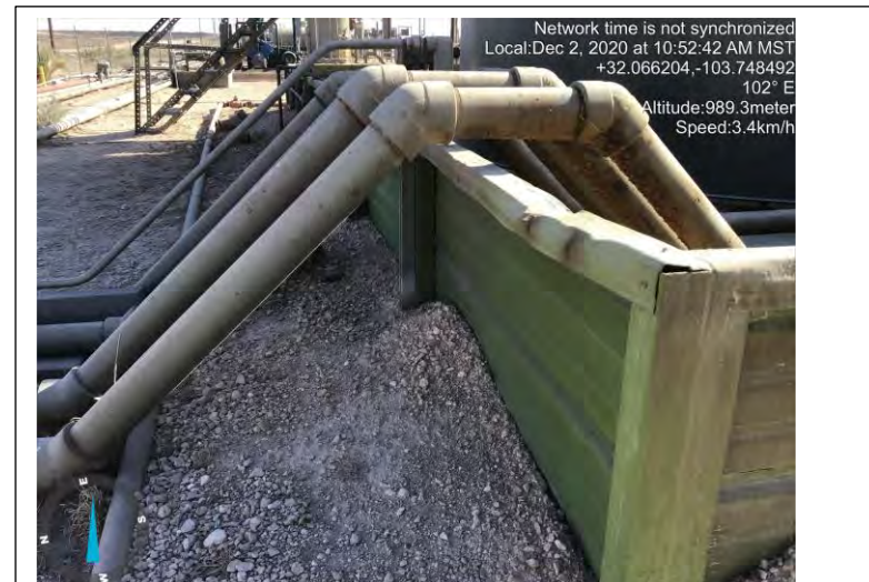
Northwest corner facing East outside
