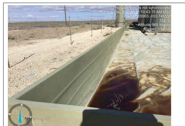
Southwest corner facing North inside
