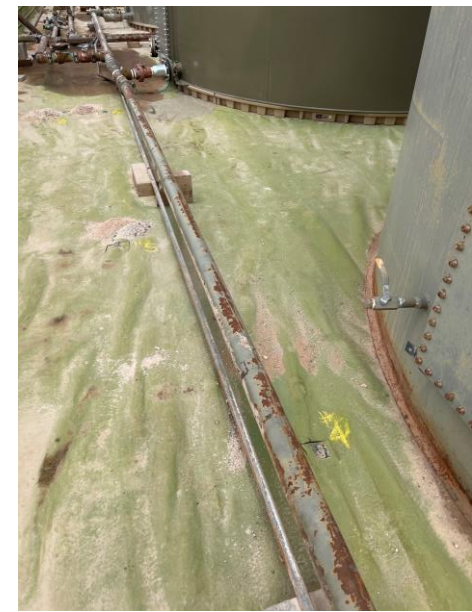
Liner Sample Point #4-facing North
