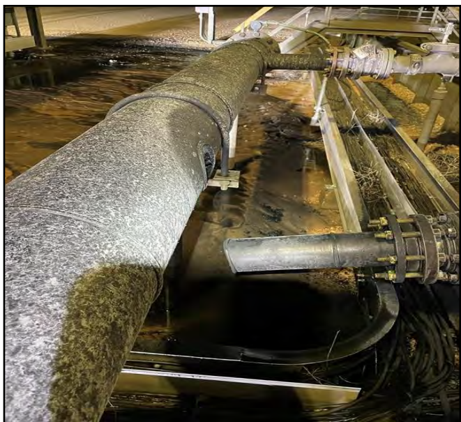
Photo of the lined containment release.
