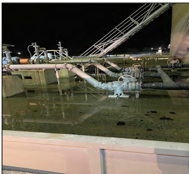
Photo of the lined containment release.
