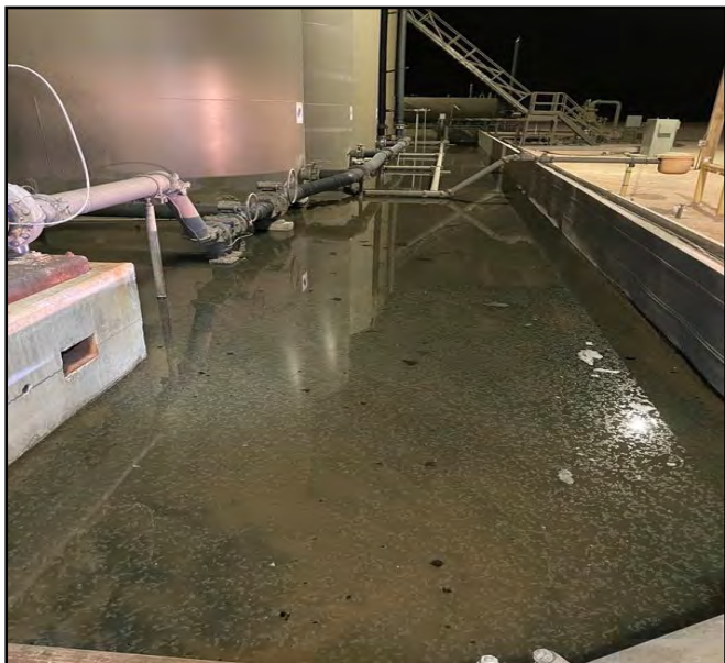
Photo of the lined containment release.
