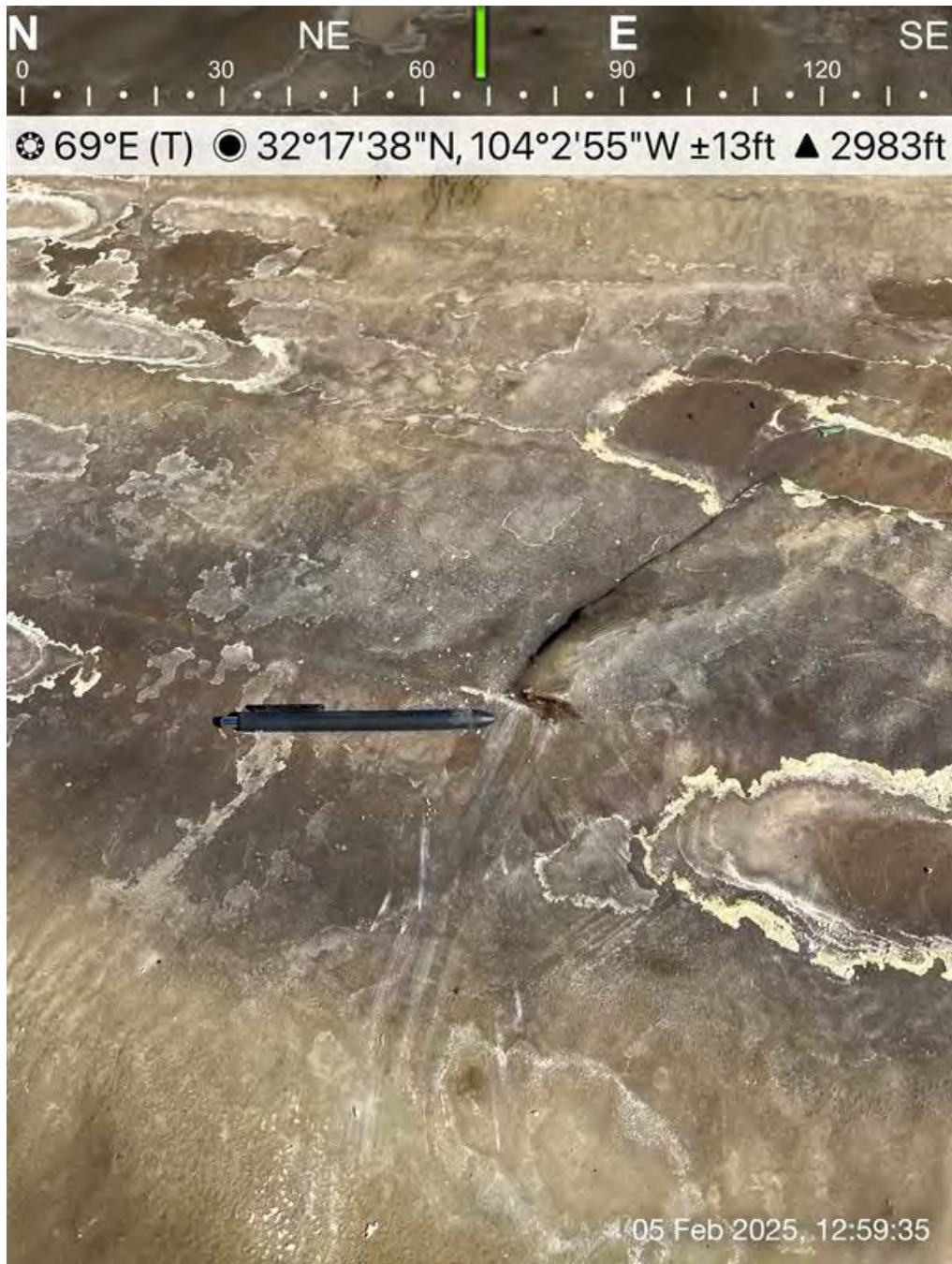
Figure 2 – Crease in Liner
