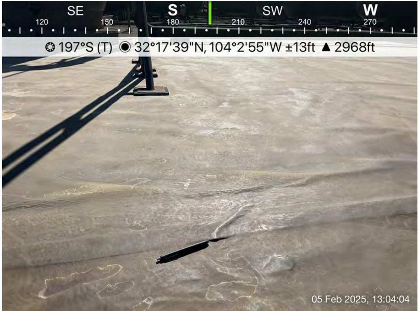
Figure 4 – Crease in liner seam
