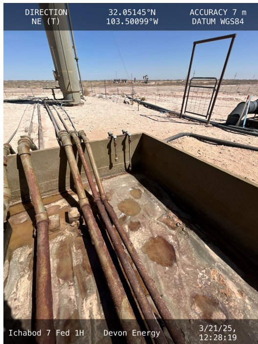
Photo 5 View of northeast corner of secondary containment. Residual fluid from power washing activities were observed.
