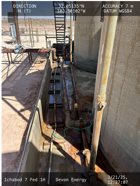
Photo 1 View of west side containment towards north. Residual fluid from power washing activities were observed.
