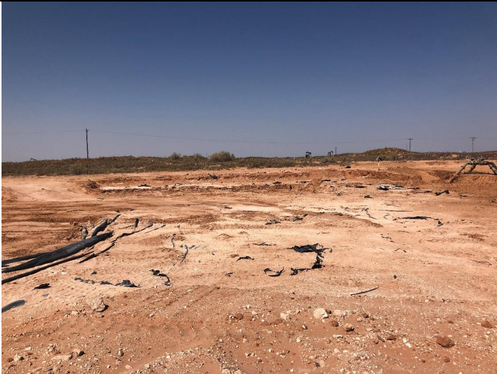
PHOTO 8: View of the excavated area and exposed liner 3 feet bgs, facing north .10/7/2020
