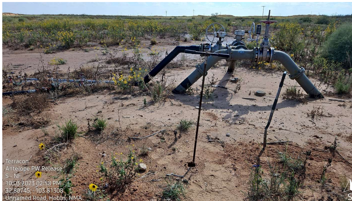
PHOTO 11: South facing view of the remediated area.
