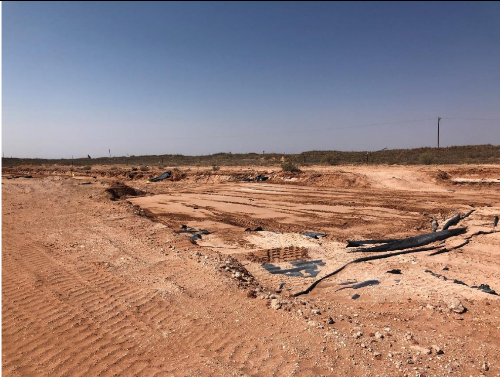
PHOTO 7: View of the excavated area and exposed liner 3 feet bgs, facing northwest .10/7/2020
