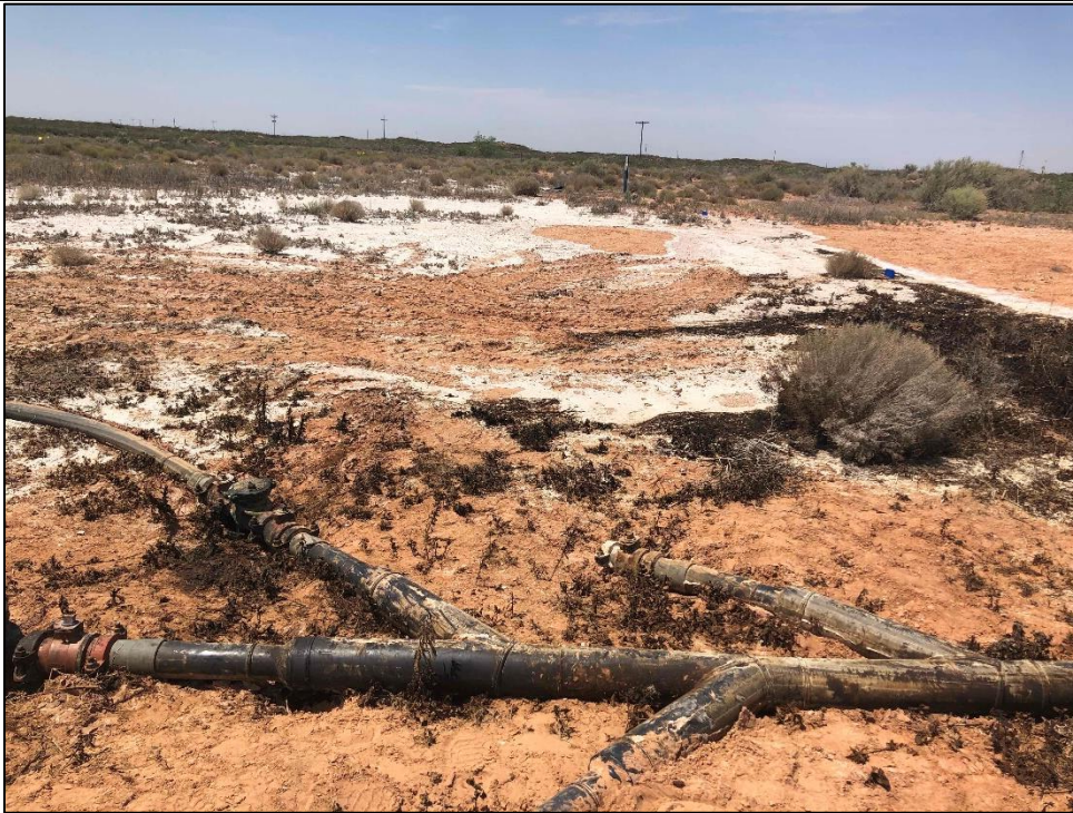
PHOTO 1: View of release point and flat topography, facing south. 6/17/2020
