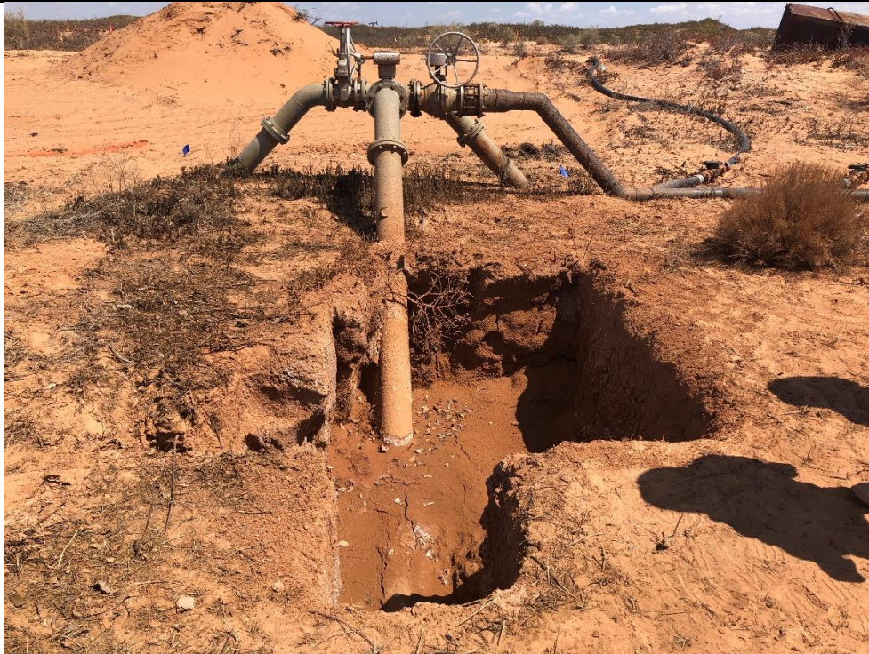
PHOTO 11: View of hydrovacted area and exposed connector, facing east .10/7/2020
