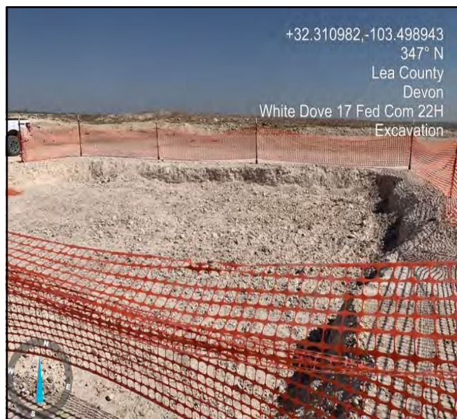
Photo during excavation facing North.
