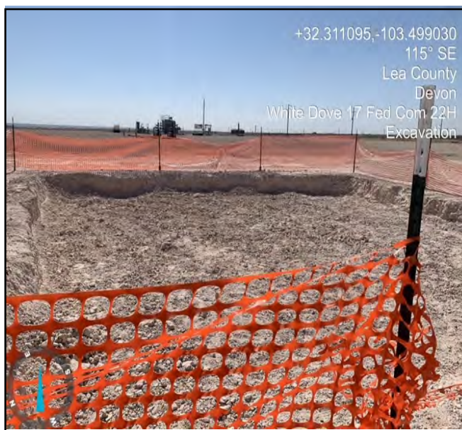
Photo during excavation facing Southeast.
