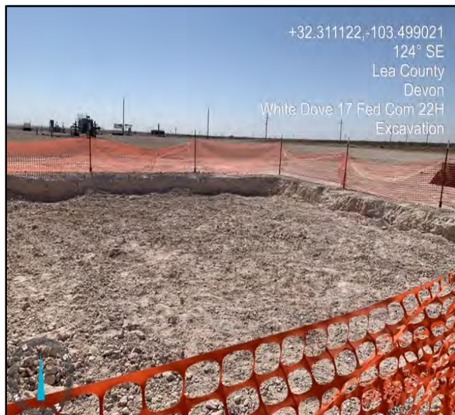
Photo during excavation facing Southeast.
