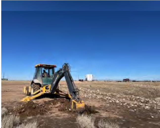
View to N of sample S-6 location.
