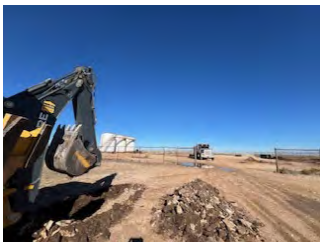
View to N of sample S-4 location.
