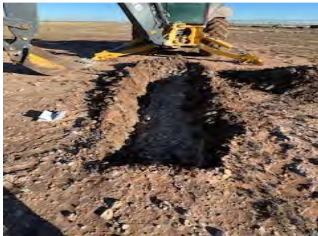
View to SW of sample S-19 location.
