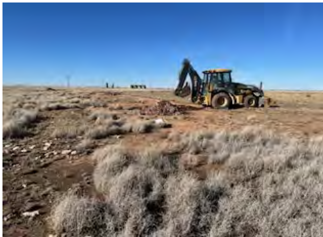
View to N of sample S-15 location.
