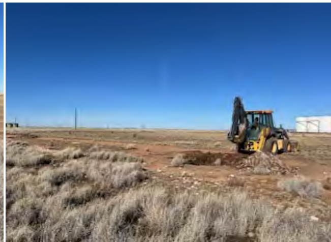
View to NE of sample S-16 location.
