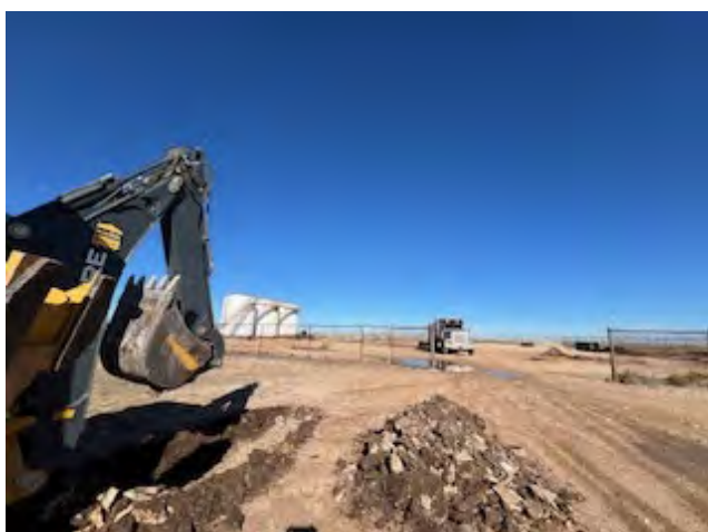
View to N of sample S-4 location.
