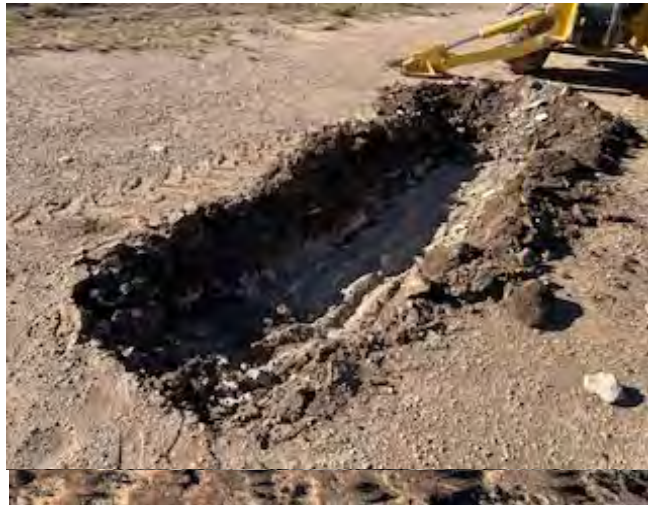
View to NE of sample S-17 location.
