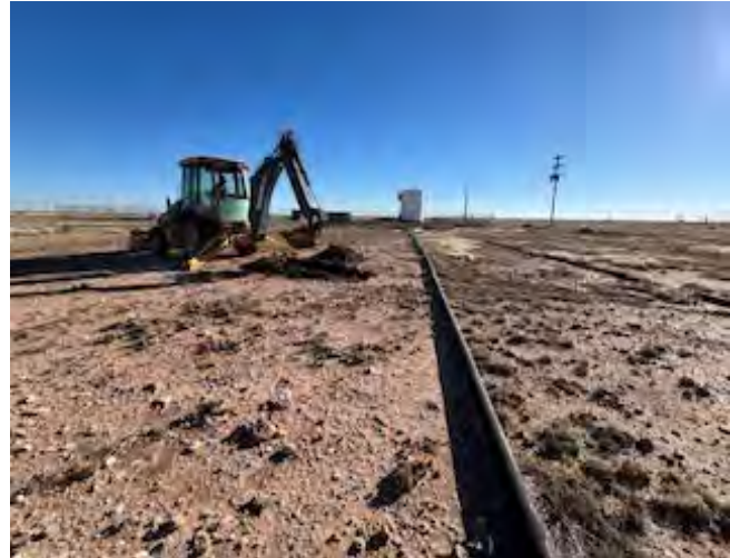
View to S of sample S-18 location.
