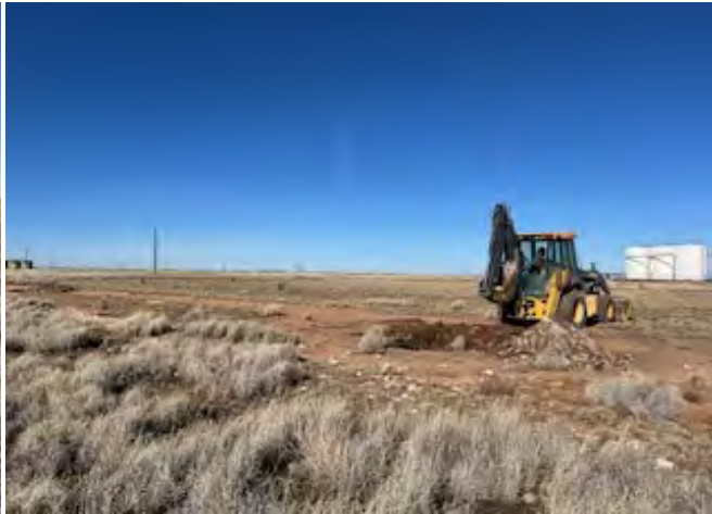
View to NE of sample S-16 location.
