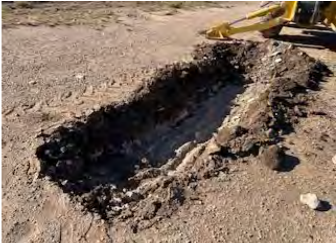
View to NW of sample S-13 location.
