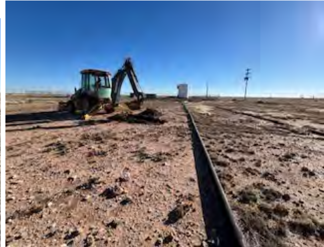
View to S of sample S-18 location.
