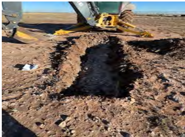
View to SW of sample S-19 location.
