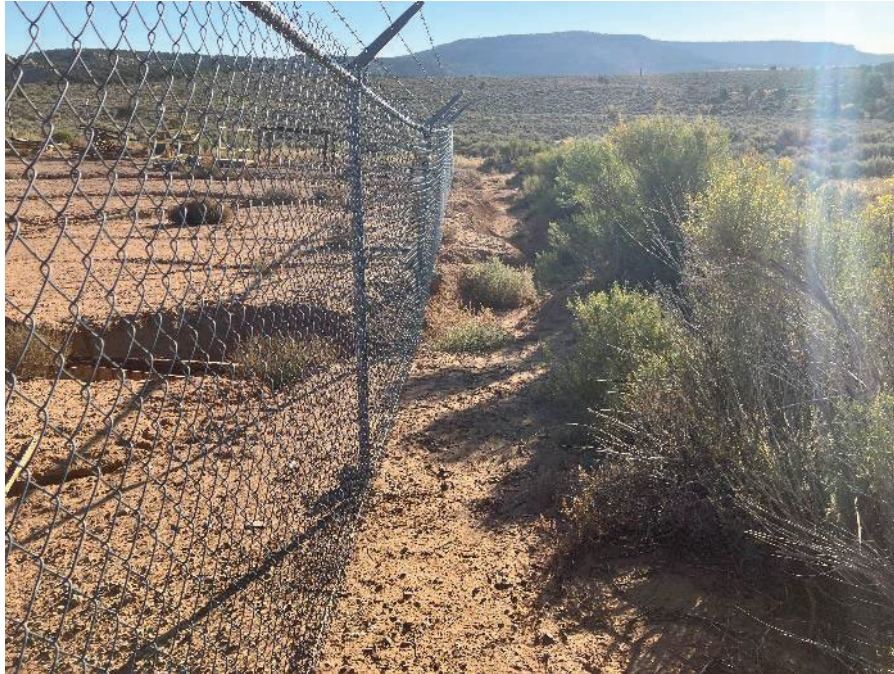
Photo 7: Erosion channel leaving facility in southeast corner.
