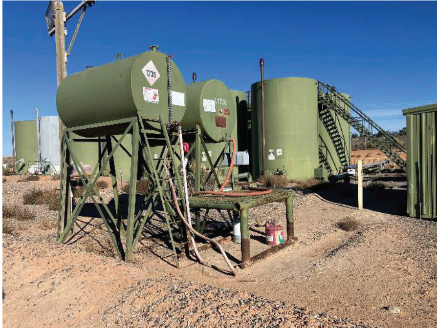
Photo 11: Tanks where containment and spill prevention need to be improved.
