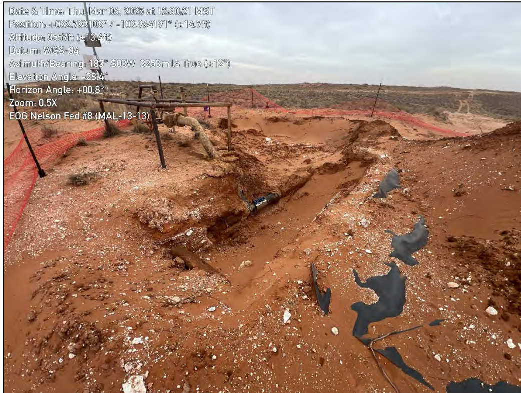
PHOTO 1: Southwestern view after initial excavation and repairs made by Kinetik. 03/06/2025
