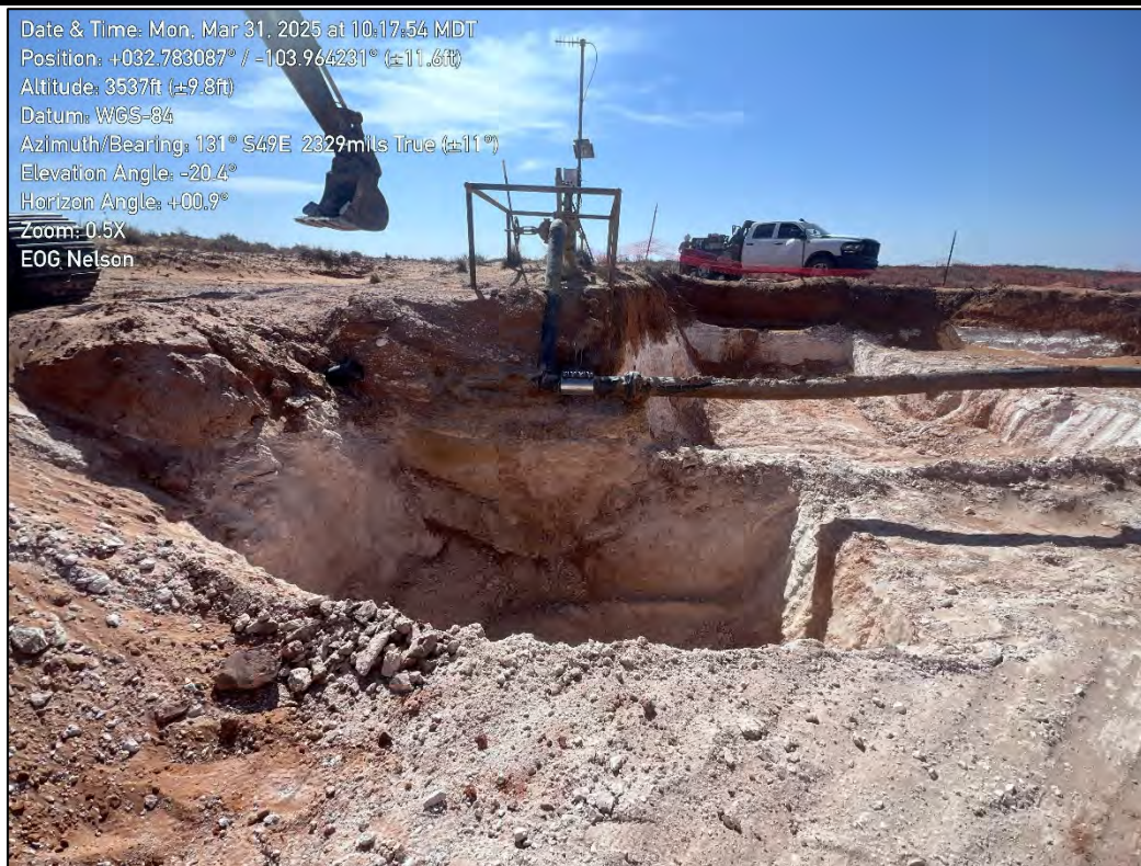
PHOTO 7: Southeastern view of excavation extent. 03/31/2025
