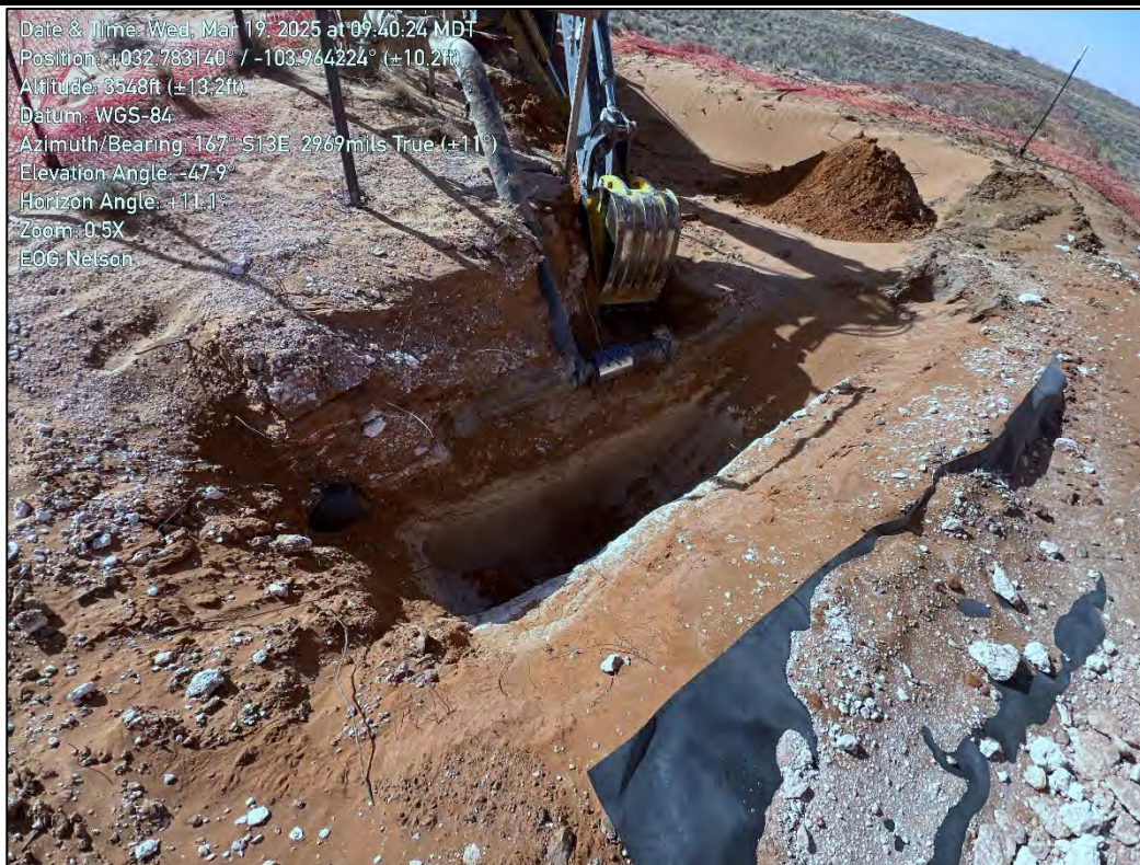
PHOTO 3: Southeastern view during delineation activities. 03/19/2025
