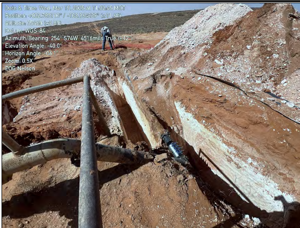
PHOTO 4: Southeastern view during delineation activities. 03/19/2025
