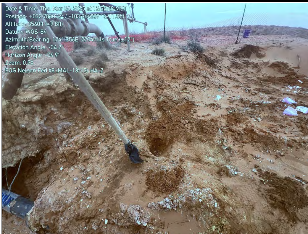
PHOTO 2: Southeastern view during delineation activities. 03/06/2025
