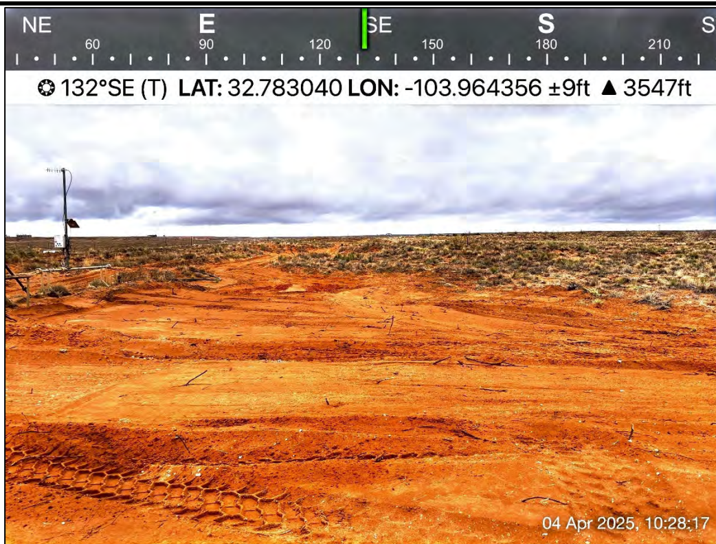
PHOTO 9: Southeastern view after restoration activities. 04/04/2025
