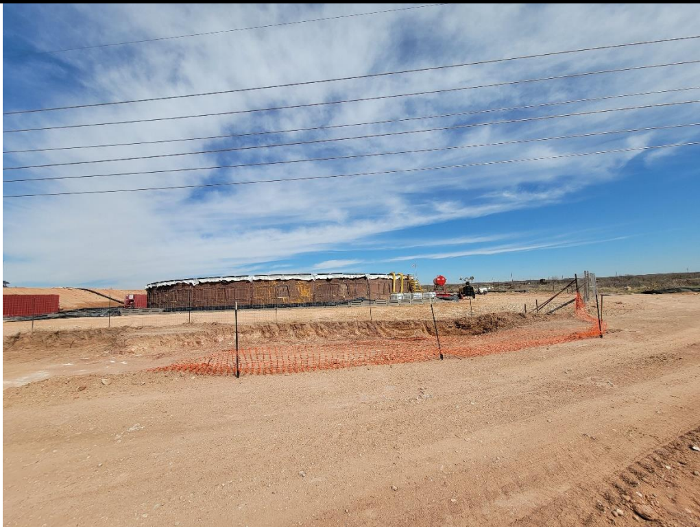
PHOTO 4: View of southern extent of the excavation.
