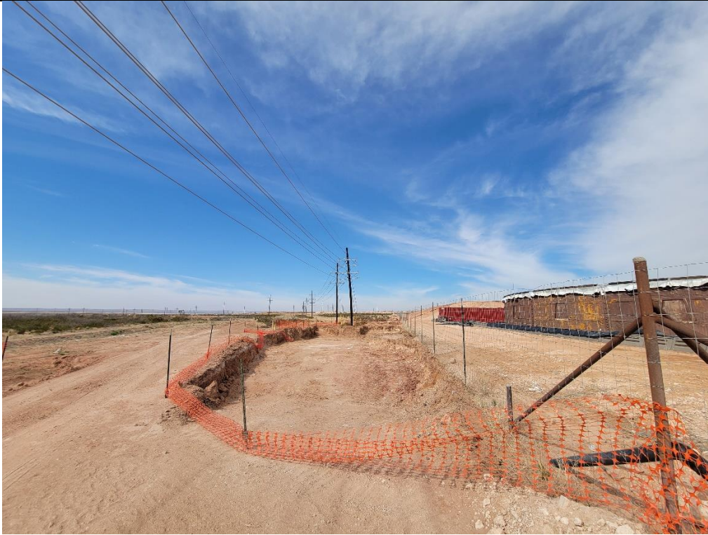
PHOTO 5: View of the excavation area facing north.
