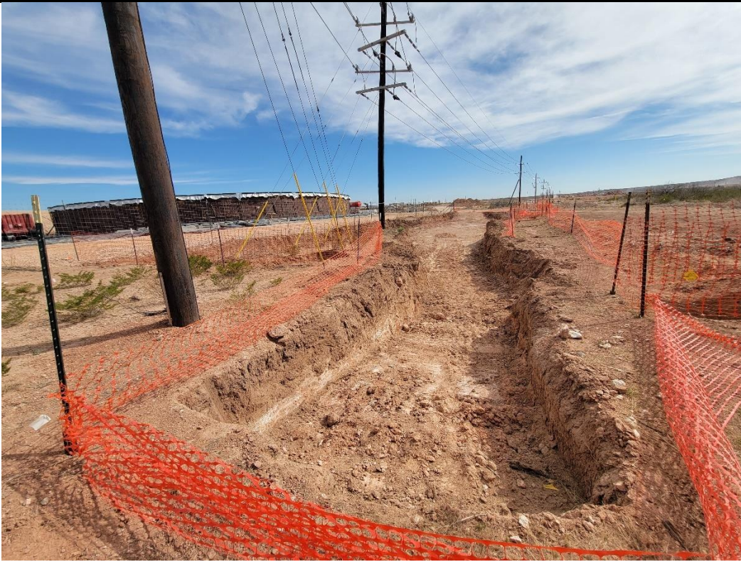
PHOTO 1: View of northern extent of the excavation.
