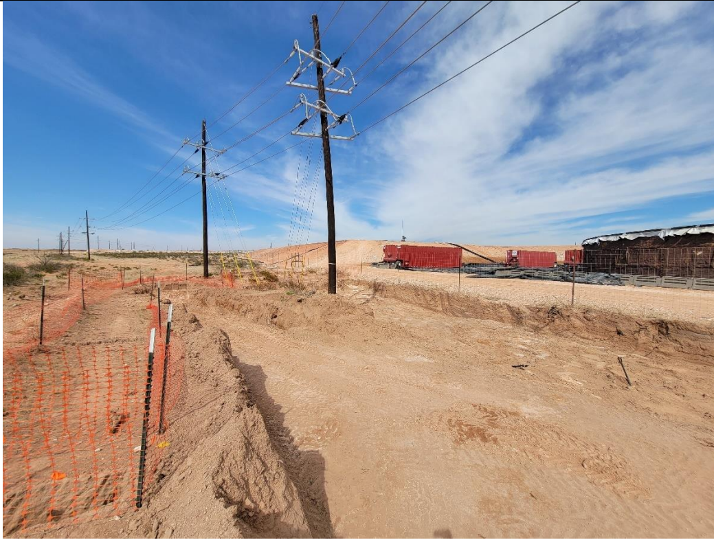
PHOTO 3: View of central excavation area.
