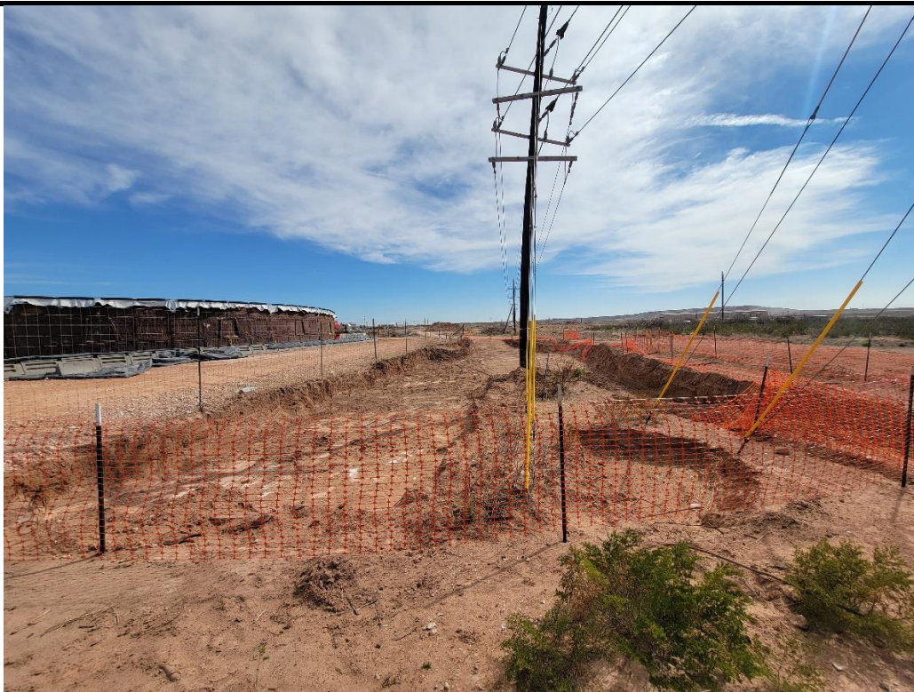
PHOTO 2: View of northern extent of the excavation.
