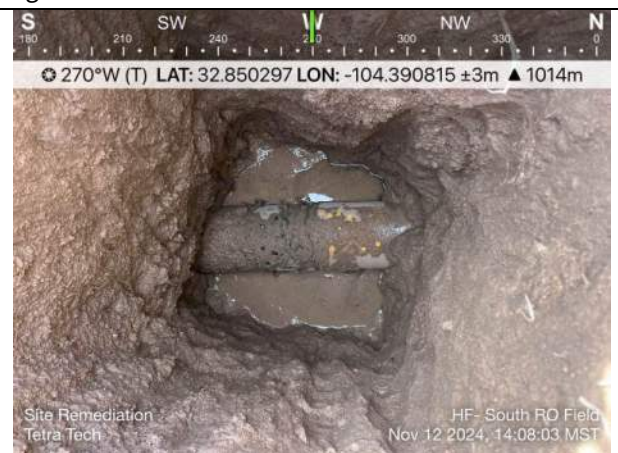
Photo 12: South RO Field, second 10-inch petroleum pipeline; location in southern portion of field; 3.5 ft bgs.
