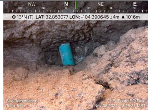
Photo 14: North RO Field, 8-inch petroleum pipeline; location in northern portion of field; 3 ft bgs.
