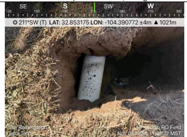
Photo 6: South RO Field, 10-inch petroleum pipeline; location in northern portion of field; 3.5 ft bgs.
