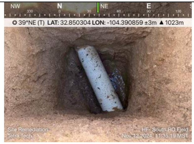
Photo 8: South RO Field, 10-inch petroleum pipeline; location in southern portion of field; 3.5 ft bgs.
