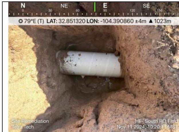
Photo 7: South RO Field, 10-inch petroleum pipeline; location in middle portion of field; 3.5 ft bgs.
