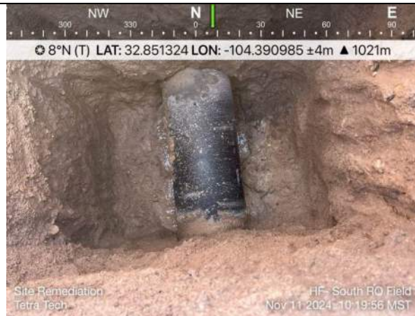
Photo 3: South RO Field, 12-inch petroleum pipeline; location in middle portion of field; 6 ft bgs.
