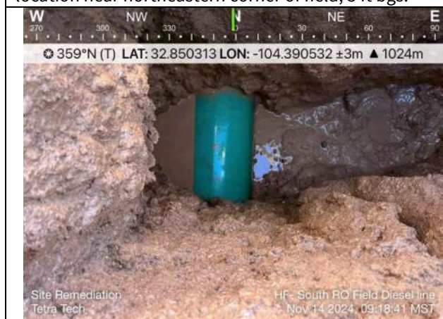
Photo 21: South RO Field, 12-inch diesel pipeline; location near southern end of field; 3.5 ft bgs.
