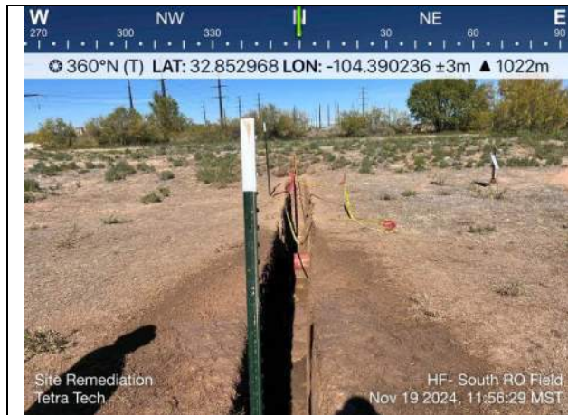
Photo 17: South RO Field, 15-inch petroleum pipeline; 20 ft long trench east of 90-degree turn inside northwestern corner of South RO field; 5 ft bgs.
