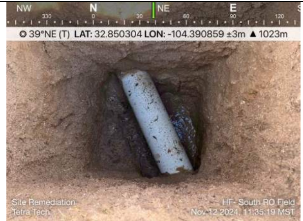
Photo 8: North RO Field, 10-inch petroleum pipeline; location in Northern portion of field; 3.5 ft bgs.
