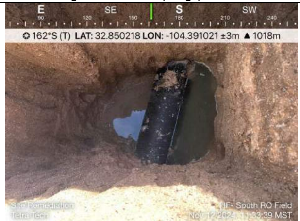
Photo 4: North RO Field, 12-inch petroleum pipeline; location in Northern portion of field; 6 ft bgs.
