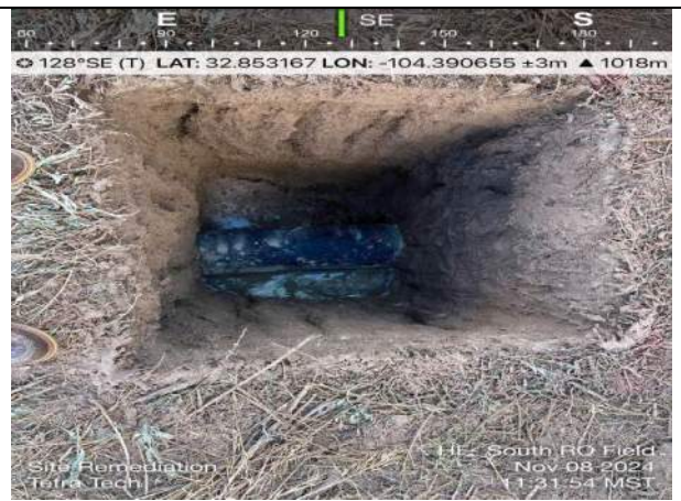
Photo 10: South RO Field, second 10-inch petroleum pipeline; location in northern portion of field; 3.5 ft bgs.
