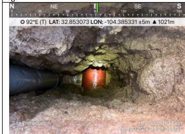
Photo 19: North RO Field, 15-inch petroleum pipeline; location near northeastern corner of field; 5 ft bgs.
