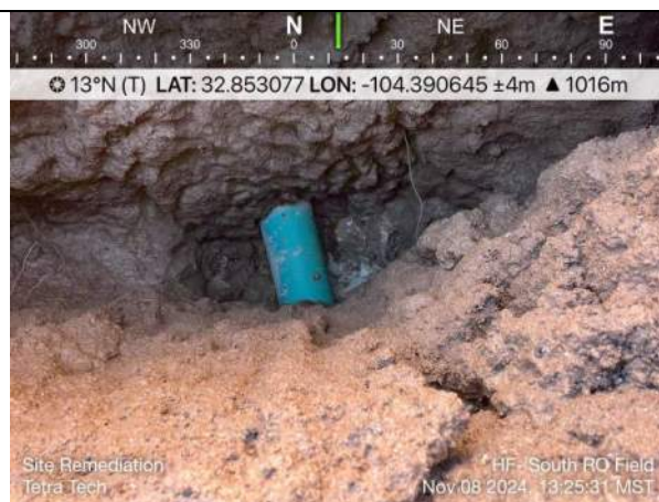
Photo 14: South RO Field, 8-inch petroleum pipeline; location in northern portion of field; 3 ft bgs.
