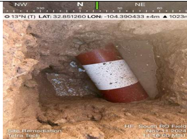
Photo 16: South RO Field, 15-inch petroleum pipeline; location in middle portion of north-south section of pipeline; 5 ft bgs.
