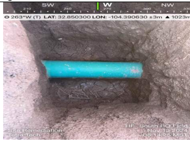
Photo 16: North RO Field, 8-inch petroleum pipeline; location in Northern portion of field; 3 ft bgs.
