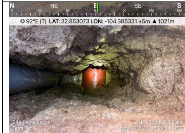
Photo 19: South RO Field, 15-inch petroleum pipeline; location near northeastern corner of field; 5 ft bgs.
