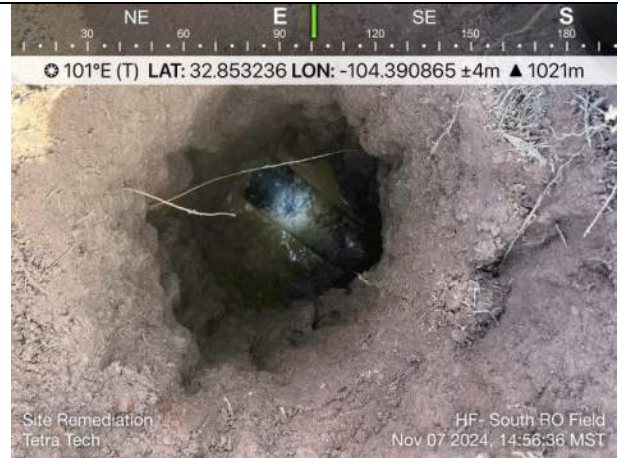
Photo 2: North RO Field, 12-inch petroleum pipeline; location in northern portion of field; 6 feet below ground surface (ft bgs).
