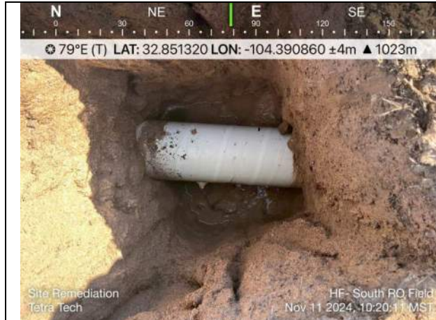
Photo 7: North RO Field, 10-inch petroleum pipeline; location in middle portion of field; 3.5 ft bgs.
