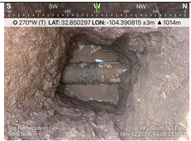
Photo 12: North RO Field, second 10-inch petroleum pipeline; location in Northern portion of field; 3.5 ft bgs.
