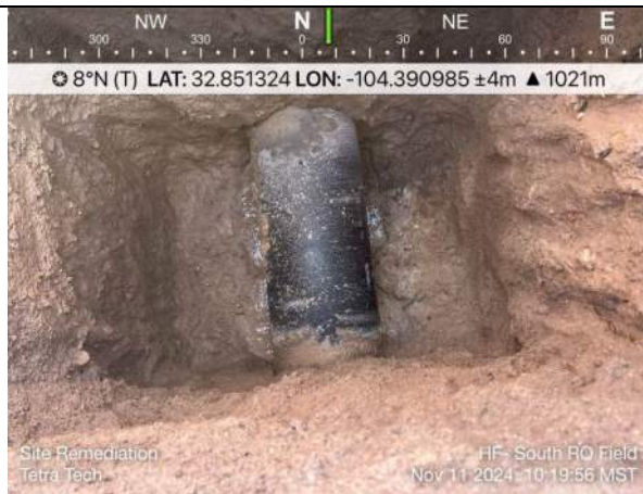
Photo 3: North RO Field, 12-inch petroleum pipeline; location in middle portion of field; 6 ft bgs.
