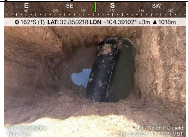
Photo 4: South RO Field, 12-inch petroleum pipeline; location in southern portion of field; 6 ft bgs.
