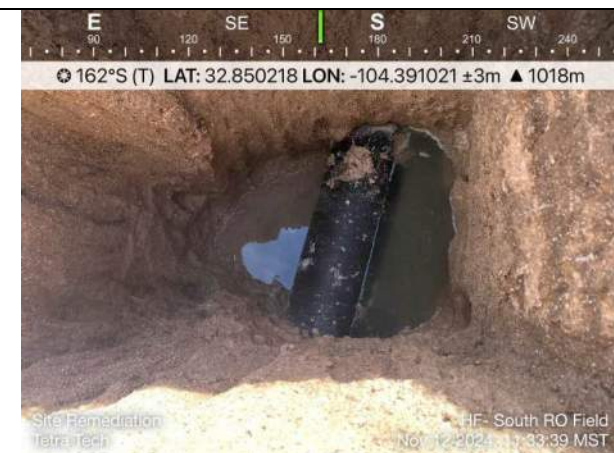
Photo 11: South RO Field, second 10-inch petroleum pipeline; location in middle portion of field; 3.5 ft bgs.
