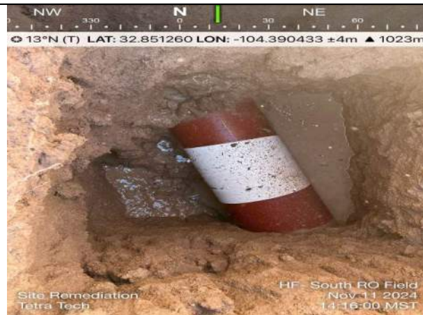
Photo 16: North RO Field, 15-inch petroleum pipeline; location in middle portion of north-North section of pipeline; 5 ft bgs.
