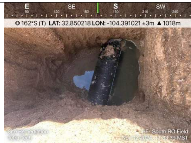
Photo 11: North RO Field, second 10-inch petroleum pipeline; location in middle portion of field; 3.5 ft bgs.
