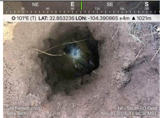
Photo 2: South RO Field, 12-inch petroleum pipeline; location in northern portion of field; 6 feet below ground surface (ft bgs).
