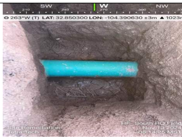
Photo 16: South RO Field, 8-inch petroleum pipeline; location in southern portion of field; 3 ft bgs.
