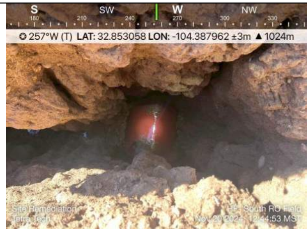
Photo 18: North RO Field, 15-inch petroleum pipeline; location on North side of northern berm approximately halfway between 90-degree elbow and eastern berm; 4.5 ft bgs.
