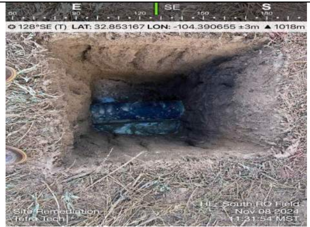
Photo 10: North RO Field, second 10-inch petroleum pipeline; location in northern portion of field; 3.5 ft bgs.
