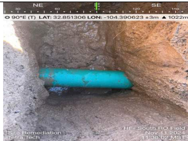
Photo 15: North RO Field, 8-inch petroleum pipeline; location in middle portion of field; 3 ft bgs.
