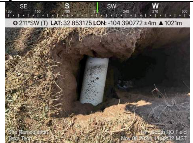
Photo 6: North RO Field, 10-inch petroleum pipeline; location in northern portion of field; 3.5 ft bgs.
