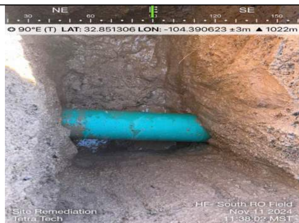
Photo 15: South RO Field, 8-inch petroleum pipeline; location in middle portion of field; 3 ft bgs.
