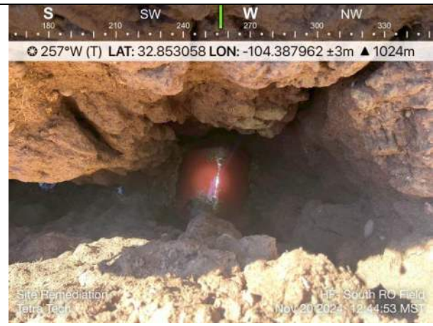
Photo 18: South RO Field, 15-inch petroleum pipeline; location on south side of northern berm approximately halfway between 90-degree elbow and eastern berm; 4.5 ft bgs.
