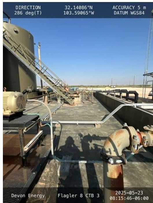
Photo 12 View of north side of secondary containment facing west.
