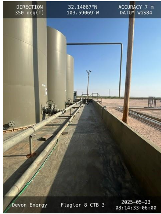
Photo 10 View of east side portion of secondary containment towards north.
