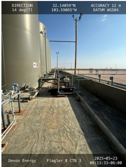
Photo 9 View of east side portion of secondary containment towards north.
