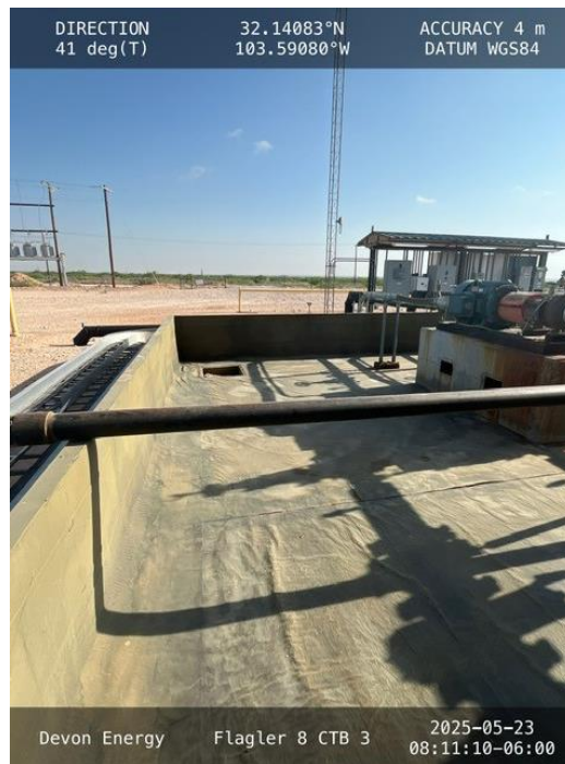
Photo 4 View of northwest corner of containment.
