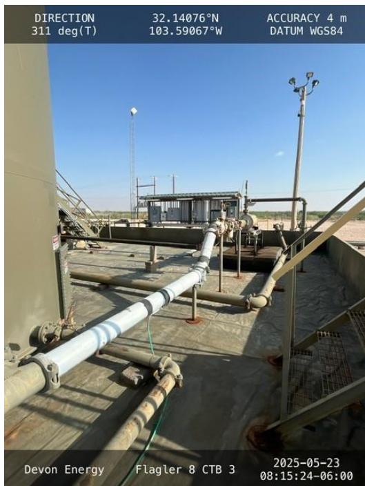
Photo 11 View of north side of secondary containment.
