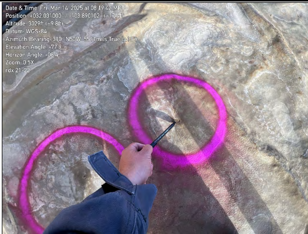
PHOTO 17: Northwestern view of failed liner integrity. 3/14/2025
