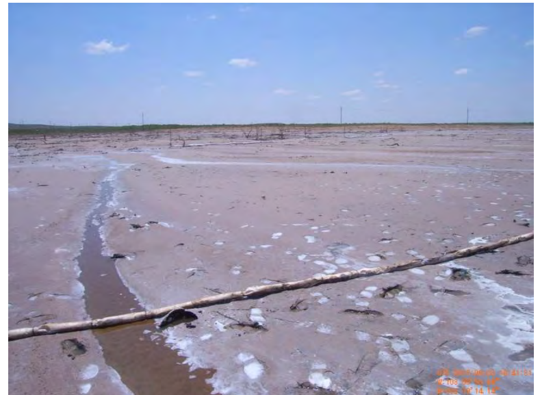
Absorbent sock placement 8/3/17
