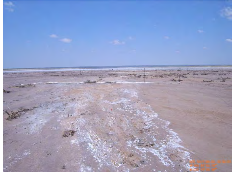
Absorbent sock placement 8/3/17
