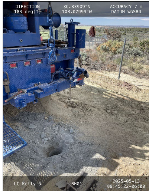
Photograph: 2 Date: 5/13/2025 Description: Complete BH01. View: South
