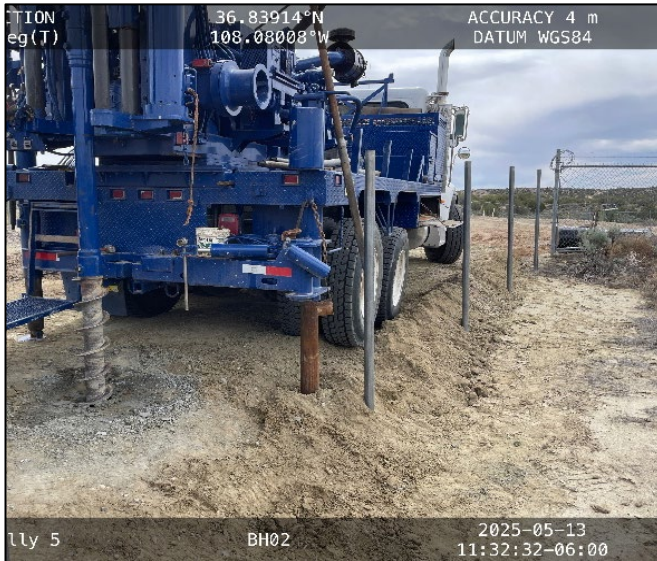
Photograph: 3 Date: 5/13/2025 Description: Drilling BH02. View: East / Southeast
