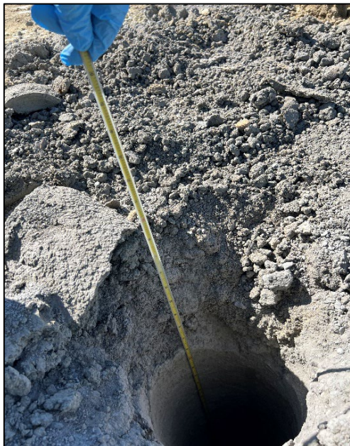
Photograph: 4 Date: 5/16/2025 Description: Open BH02 with total depth 54' BGS and no water reading on interface probe
