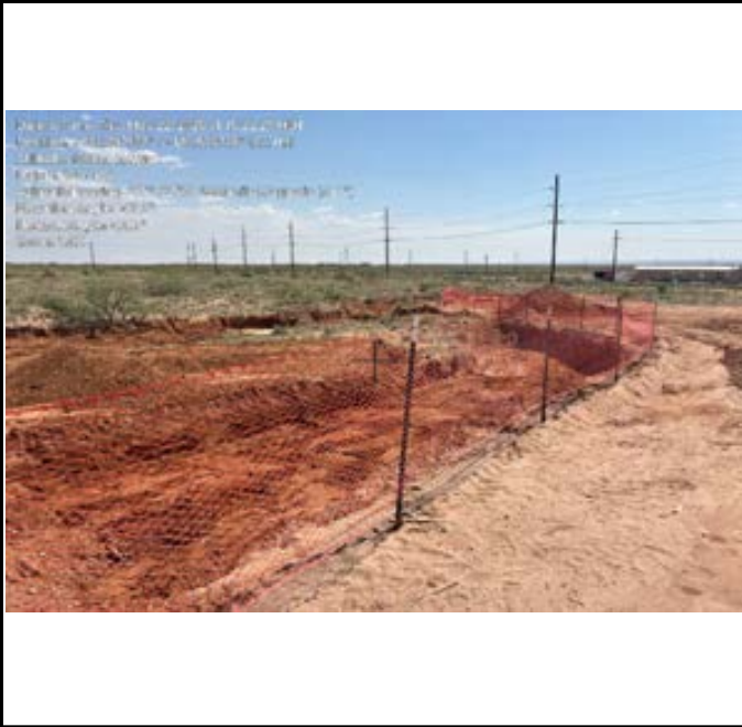
Photograph: 3 Date: 5/22/2025 Description: Excavation activities; near FS15 View: Southwest
