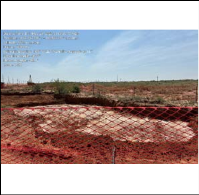
Photograph: 4 Date: 5/23/2025 Description: Excavation activities; near FS21 View: Southeast
