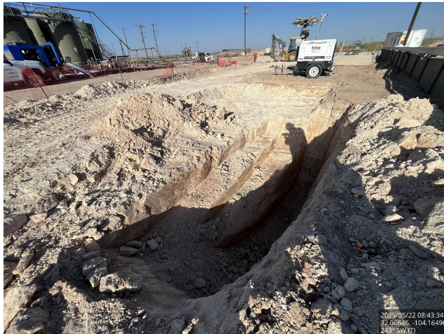
Eight foot excavated area (benched), viewing southwest.
