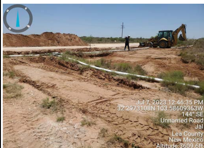
Photograph: 4 Date: 7/7/2022 Description: Excavation activities View: East
