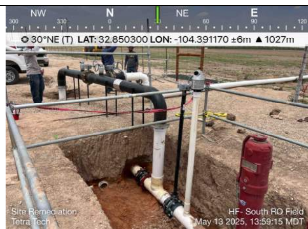
Photo 6: Valve and meter run being constructed west of South RO field.
