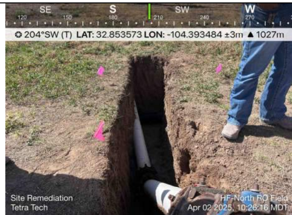
Photo 2: Connection of irrigation distribution piping to source in North RO field.
