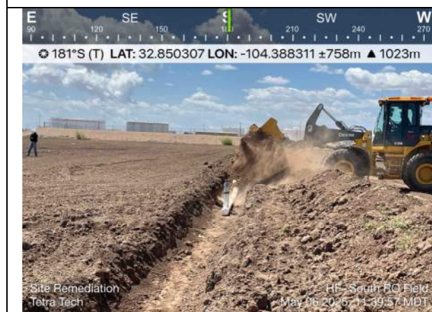
Photo 5: Backfilling irrigation distribution piping trench in South RO field.
