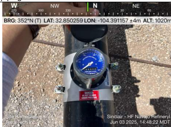
Photo 9: Flowmeter on irrigation piping run.
