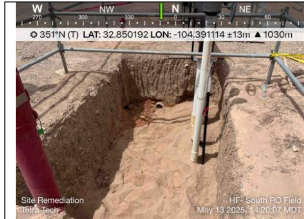
Photo 7: Initial backfill of piping run. Piping in foreground leads to process water tank. Note the firewater system is separate from the irrigation piping.
