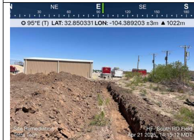
Photo 3: Trench for irrigation distribution piping in South RO field.
