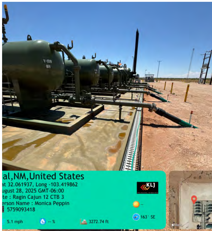
West side of containment facing south.
