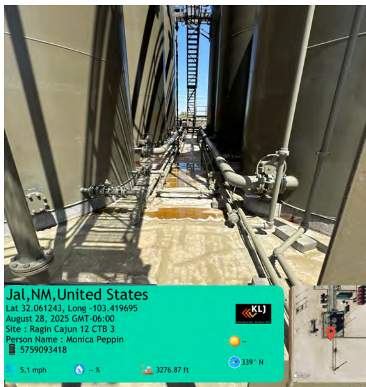
Liner between tanks facing north.
