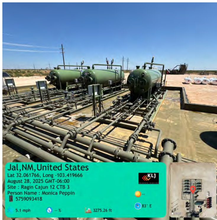
Northeast corner from mid area.
