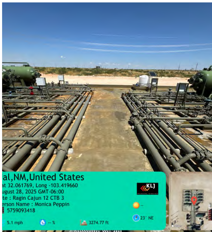
Facing North from mid area of containment.
